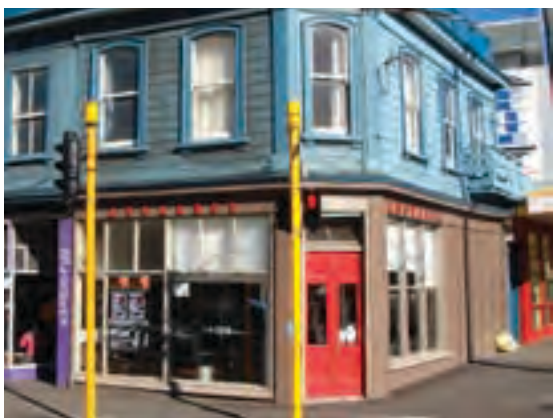
Character building on corner of Adelaide Road and Rugby Street (2008)
