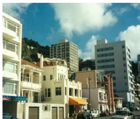
Side elevations visible from the street
