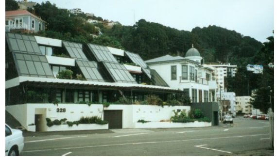
“Stepped” building form is not typical of the area
