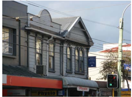
Upper level windows and parapets
