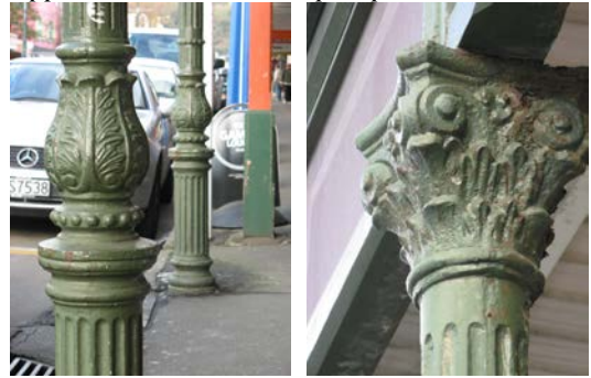
Detail of cast iron veranda posts
