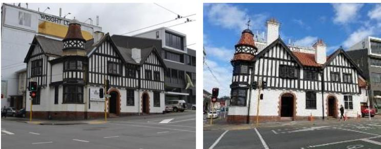
**Figure 49.** *Parts of the chimneys at 200 Willis Street were removed in the early 20th century. The remaining unreinforced masonry above roof level was removed in c.2018, and the chimneys were reinstated in as lightweight replicas. The image to the left shows the building in previous years, the image to the right shows the completed works. (Photos: Wellington City Council (left 2015) (right 2021))*
