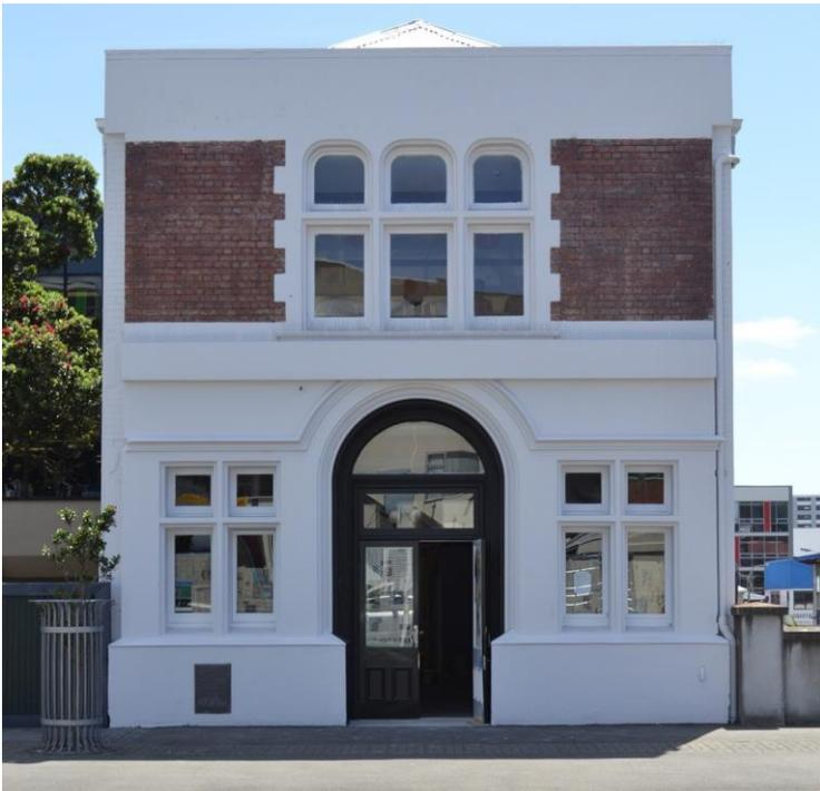
**Figure 28.** *30 Arthur Street was relocated to allow for the construction of Karo Drive. It has been restored, strengthened and returned to a sustainable long-term use. (Photo: Wellington City Council, 2015)*
