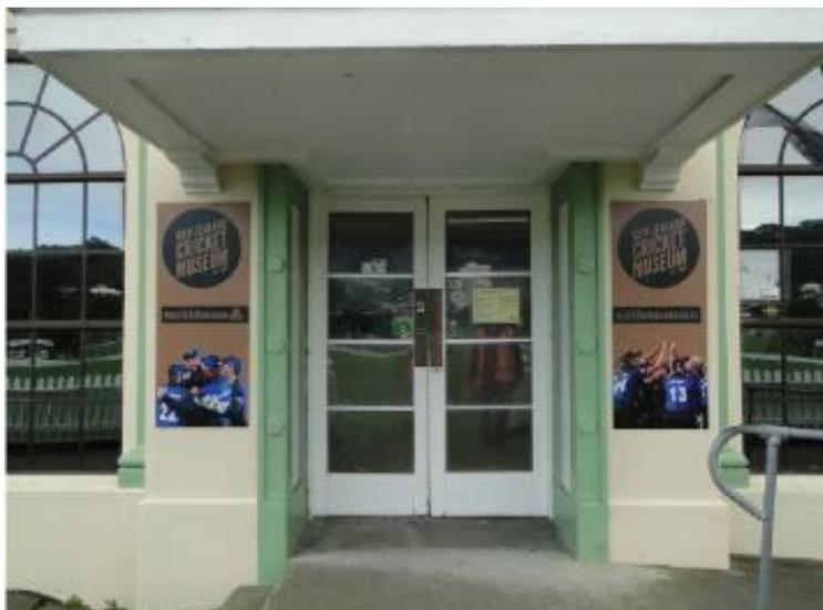
**Figure 46.** *Before - The refurbishment of the Basin Reserve Museum Stand included the removal of modern doors that were in poor condition. (Photo: Roger Shard, 2017)*
