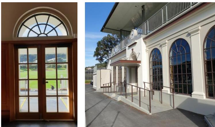
**Figure 47.** *After - The non-heritage doors were replaced with new timber joinery to match the original drawings from 1924. The door leaves have been adjusted to meet requirements for accessibility. A second ramp has been added to make the entrance symmetrical, and the handrails updated. (Photos: Wellington City Council, 2020)*
