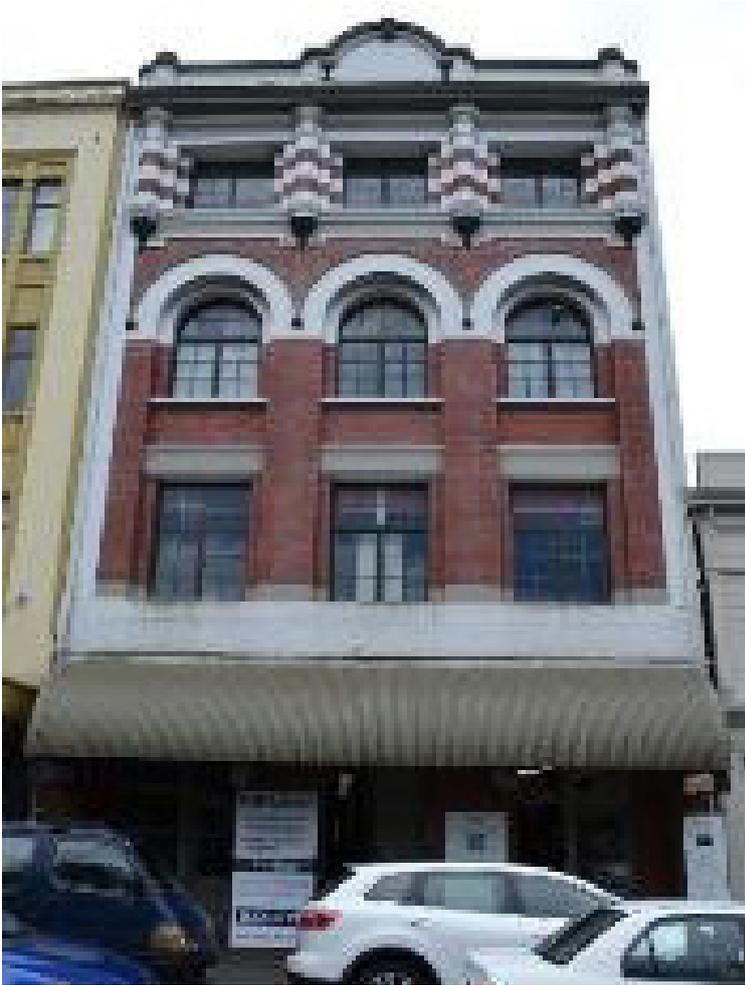
**Figure 38.** *The former Cadbury's Building at 60 Ghuznee Street, Wellington was strengthened in 2017. There are new internal reinforced concrete columns, steel cross bracing, and concealed stainless steel in the decorative columns on ground and third floors. The parapet has been restrained by a steel frame that is fixed back to the existing structure.*
