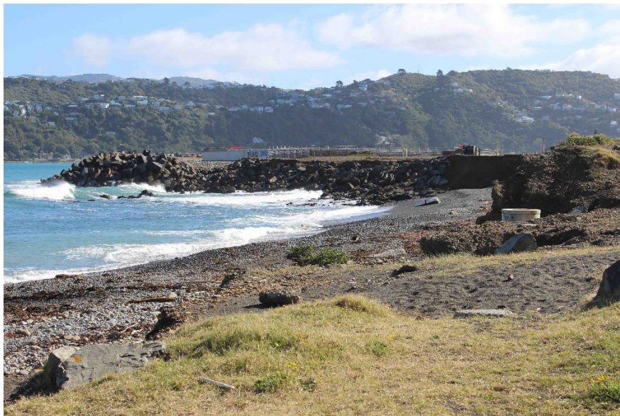
Figure 8 Wellington Airport southern seawall and Mōa Point Sewage Pipe Long Outfall
