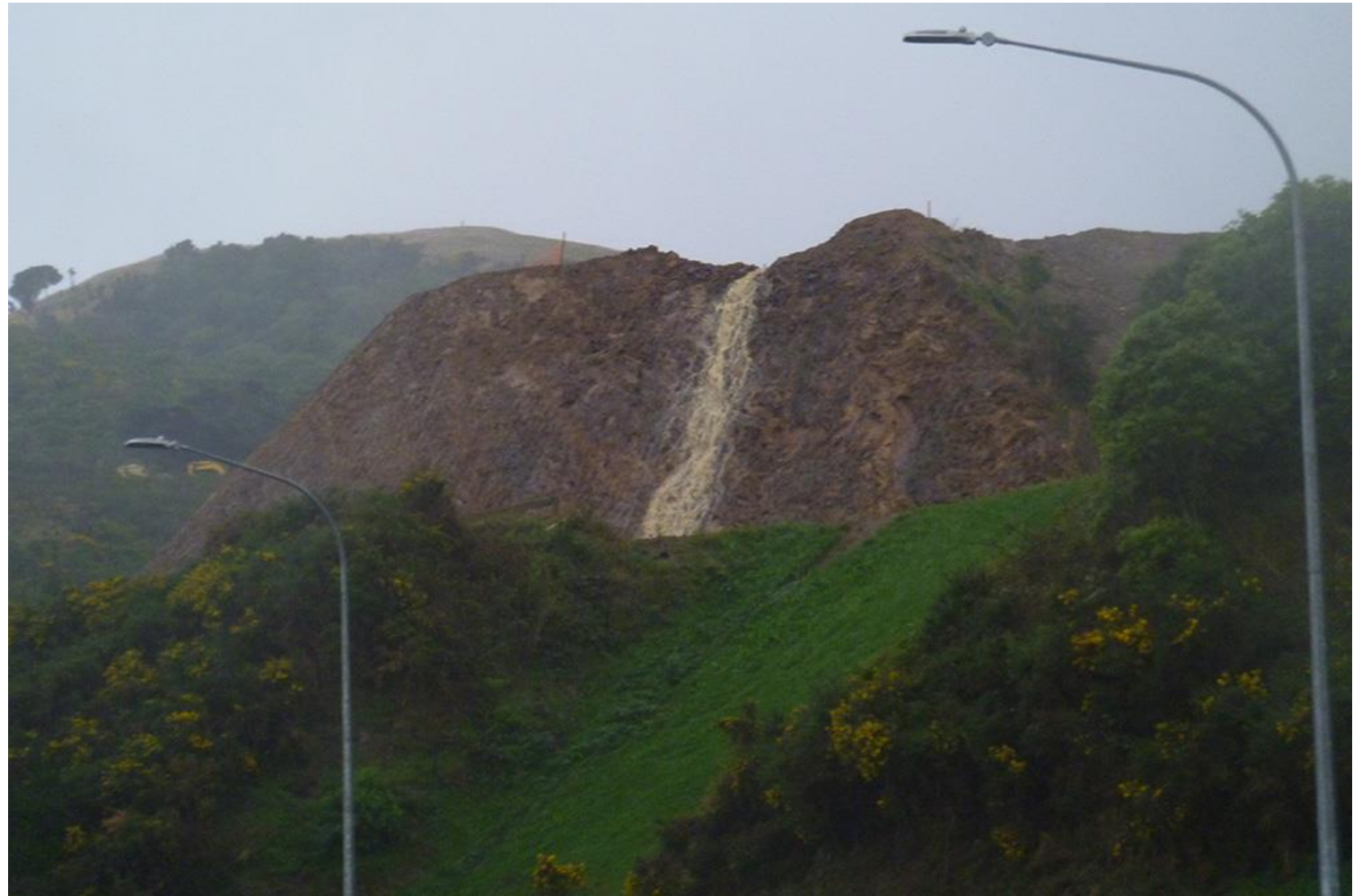
Reedy Block phase 2 during rainstorm
