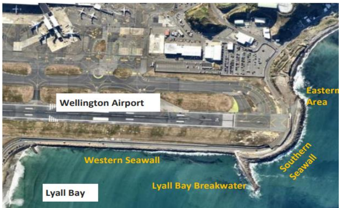
Figure 1: Seawall Structures Lyall Bay
