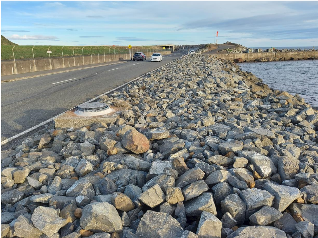
Photo 7: Moa Point Road – crest of western seawall.
