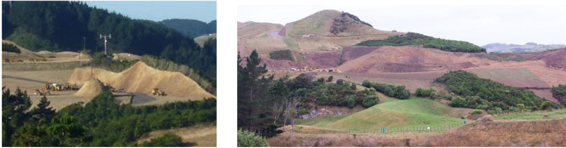
Fig 6 Earthworks in the Reedy Block
