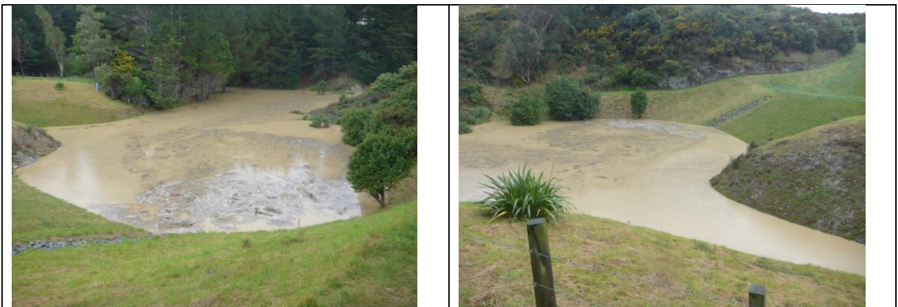
Fig 7 Stebbings Dam 2015, Seton Nossitor Dam 2020 and Debris Arrestor
