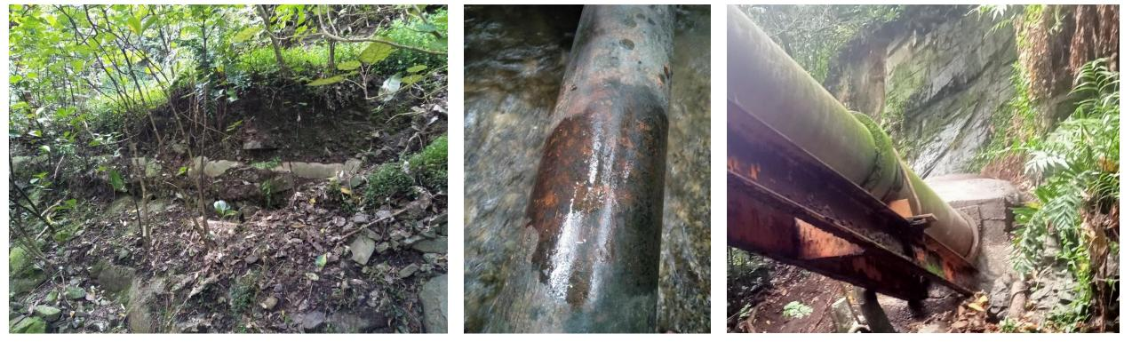
The waste water pipe has a high risk rating in the Wellington Water(WW), operational risk register and has been highlighted to WW Service planning as *in the event of failure it is unlikely that the pipeline will be able to be repaired, reconstructed or rehabilitated in the existing location due to safe access.*
