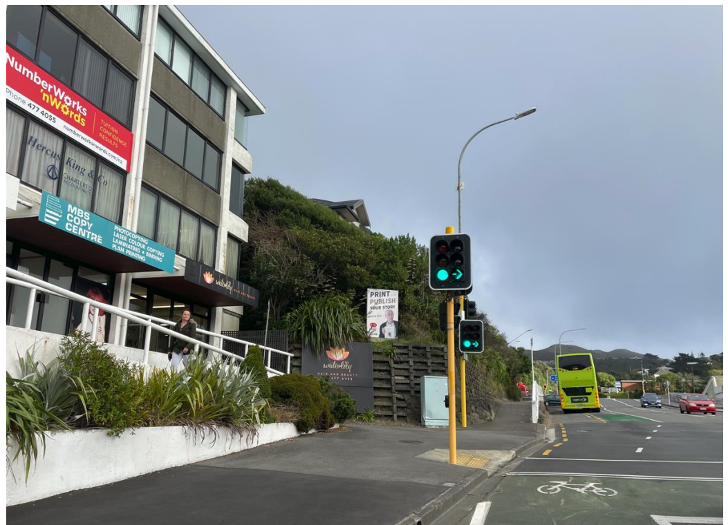
Figure 6 – View along Broderick Road looking west illustrating tallest part of retaining structure where an active frontage is recommended.
