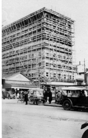
Figure 6 Hope Gibbons building under construction: National Library NZ PAColl-0125-01 (1924-1927)
