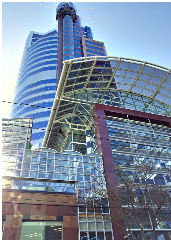
Figure 15 Corner effects of an isolated building are mitigated by the rounded planform, Boulcott Street, Wellington
