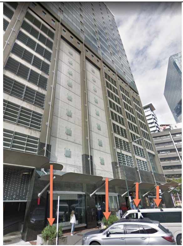
Figure 32 "Hamilton Chambers" Lambton Quay, Wellington, NZ. Proposed tree wind shelter never grew successfully. Now reduced to shrubs that grow but provide none of the promised shelter
