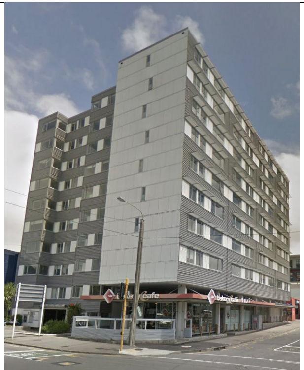
Figure 23 Example from Wellington of divided flows to reduce the problems at the foot of buildings by increasing the porosity of the building - slot through the building <1m high at first floor above retail
