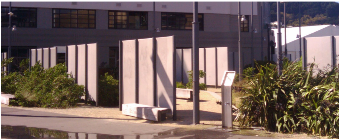
Figure 51 Porous metal screens enabling wind hardy plants to grow beside the harbour in Wellington, New Zealand
