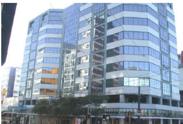
Figure 16 Chamfered corners of the tower reduce the impact on the wind of a broad flat wall, and are simpler to build than a curved planform; also open first floor car parking diverts wind flow above pedestrians. Victoria St, Wellington
