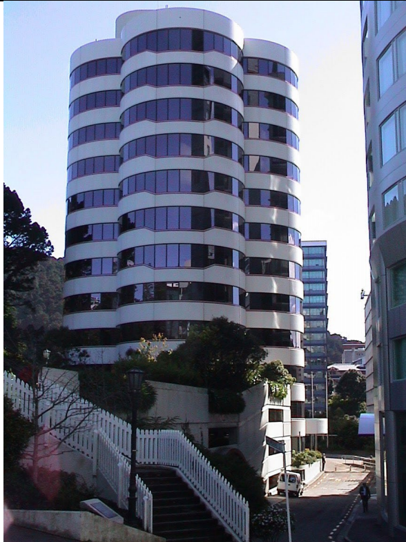
Figure 14 Corner effects of an isolated building are mitigated by 'cloud' plan shape, Bowen Street, Wellington
