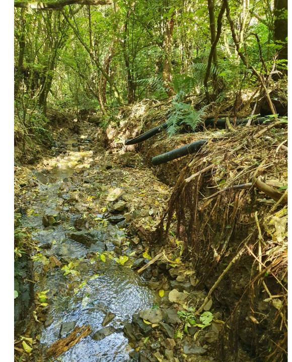
Poor stormwater management: erosion of Waste Water pipe in Tyers Stream Reserve
