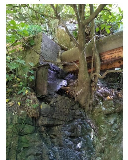
Sewage fungi due to significant waste water (sewage) leaks into Tyers Stream. Current pipe is beyond capacity.
