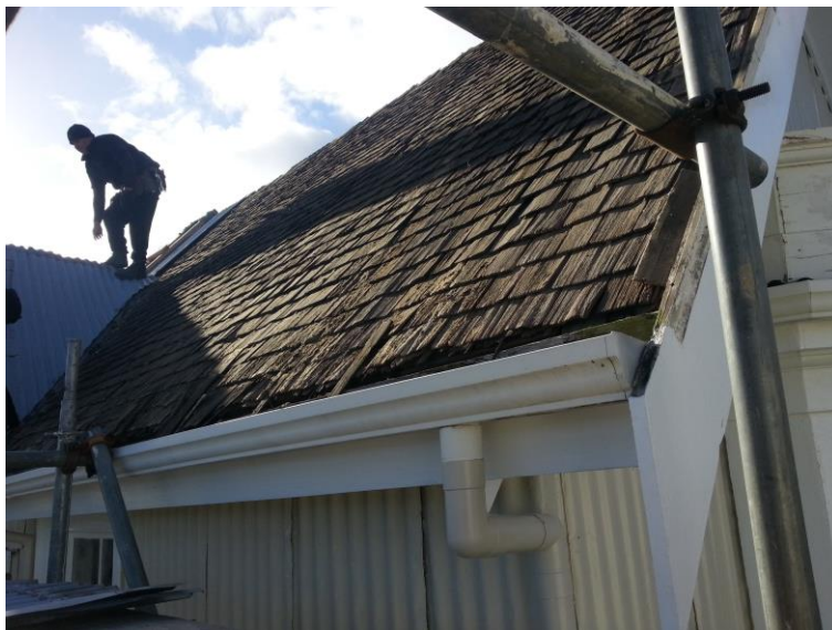
Early shingle tiles under corrugated iron, N Naus, 2013
