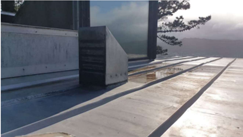
Roof at 28 Robieson Street (Photo: M Keir 2022).
