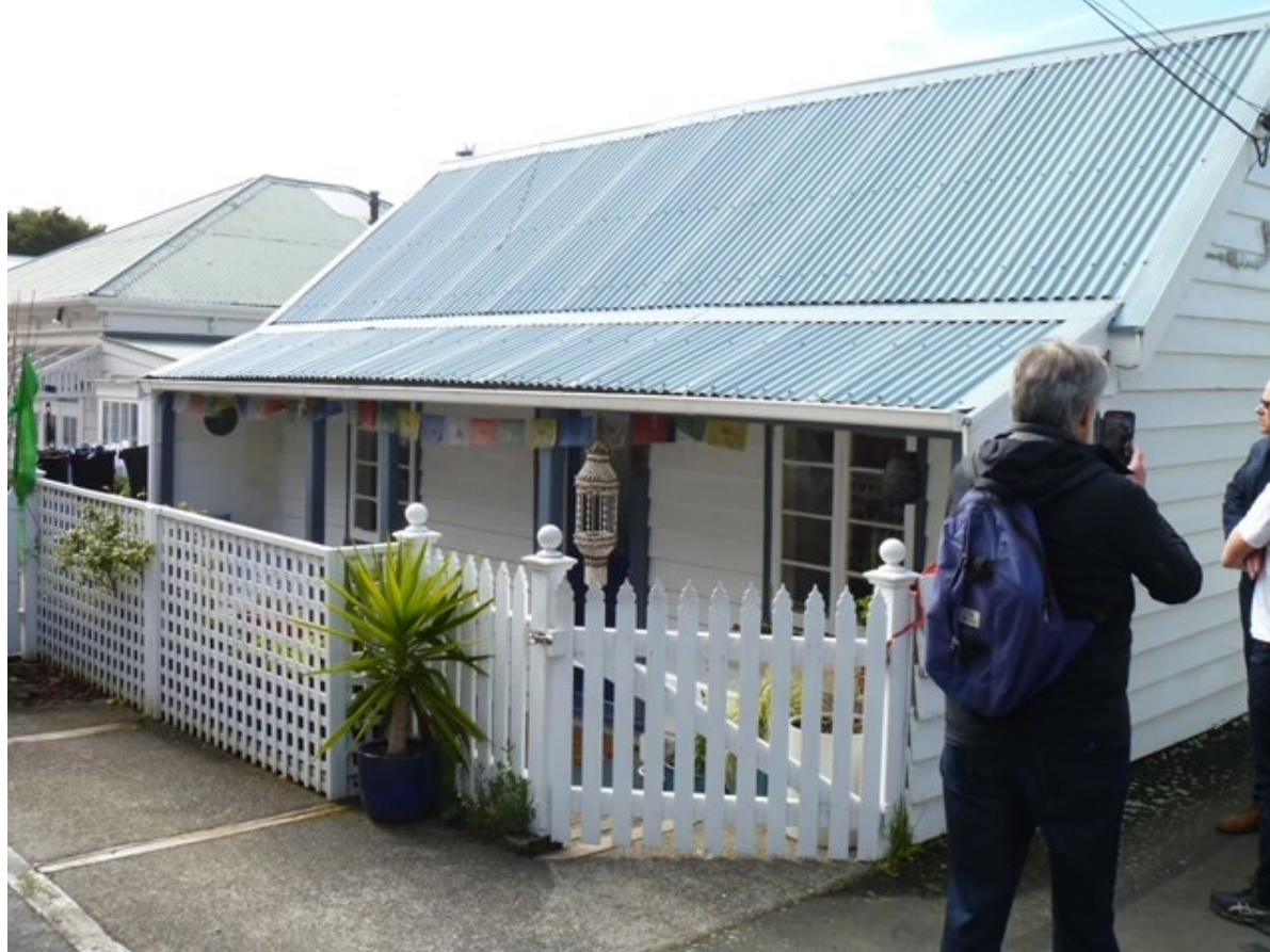
5 Torless Terrace, Thorndon (1859) – oldest house in Thorndon - add to SCHED 1
