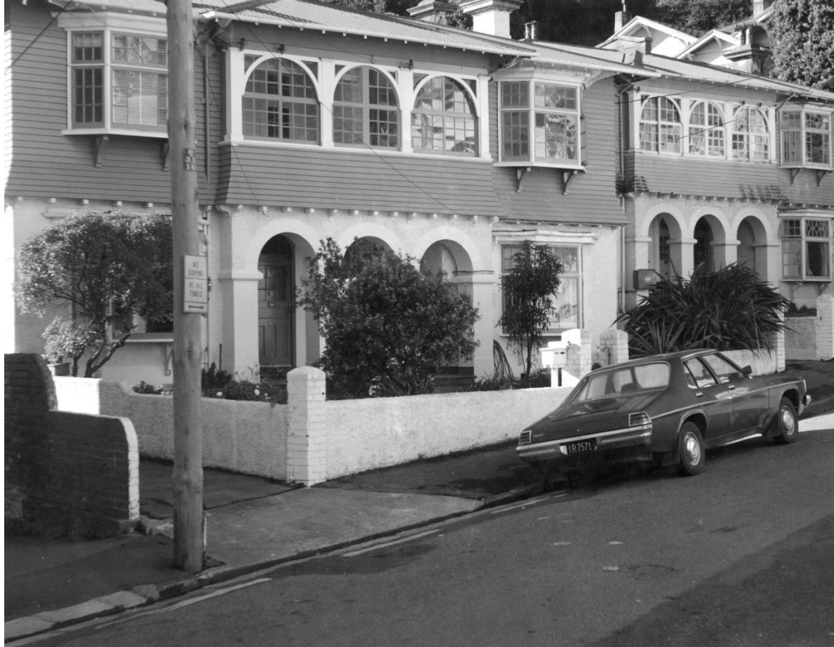
a) Wilkinson holiday flats at 5-7 and 9-11 Grass Street (1923)
