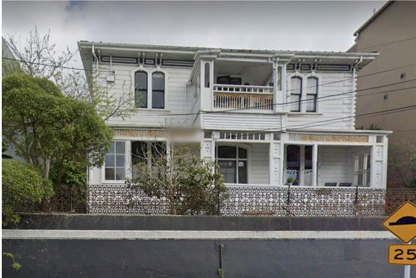
c) Samuel Brown House at 22 Hanson Street (1880)
