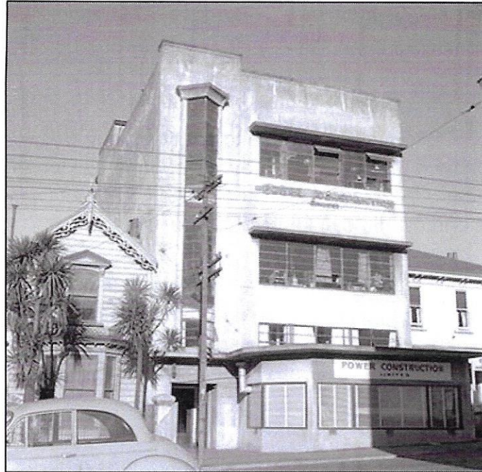
233-235 Willis Street, three storey commercial building 1960, Power Construction Ltd, 903-q (sheet 1863a), Wellington City Council Archives.
