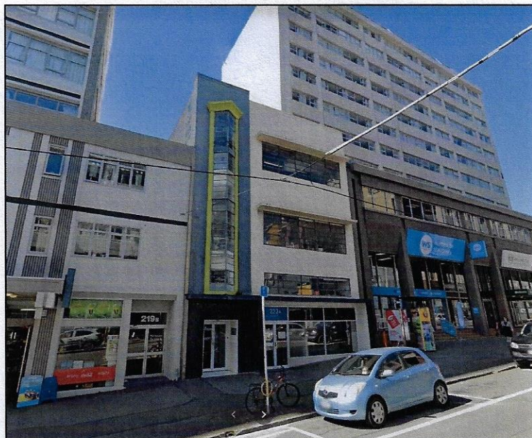
233 Willis Street, 180 Victoria Street. Google Street View 2020.
