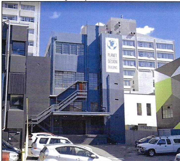
Rear of Building, 180 Victoria Street. Google Street View 2020.
