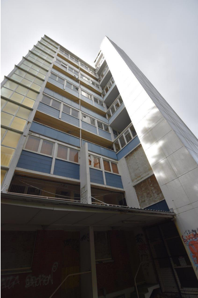
Figure 11: Rear (west) elevation showing stairwell and lift tower at northern end.
