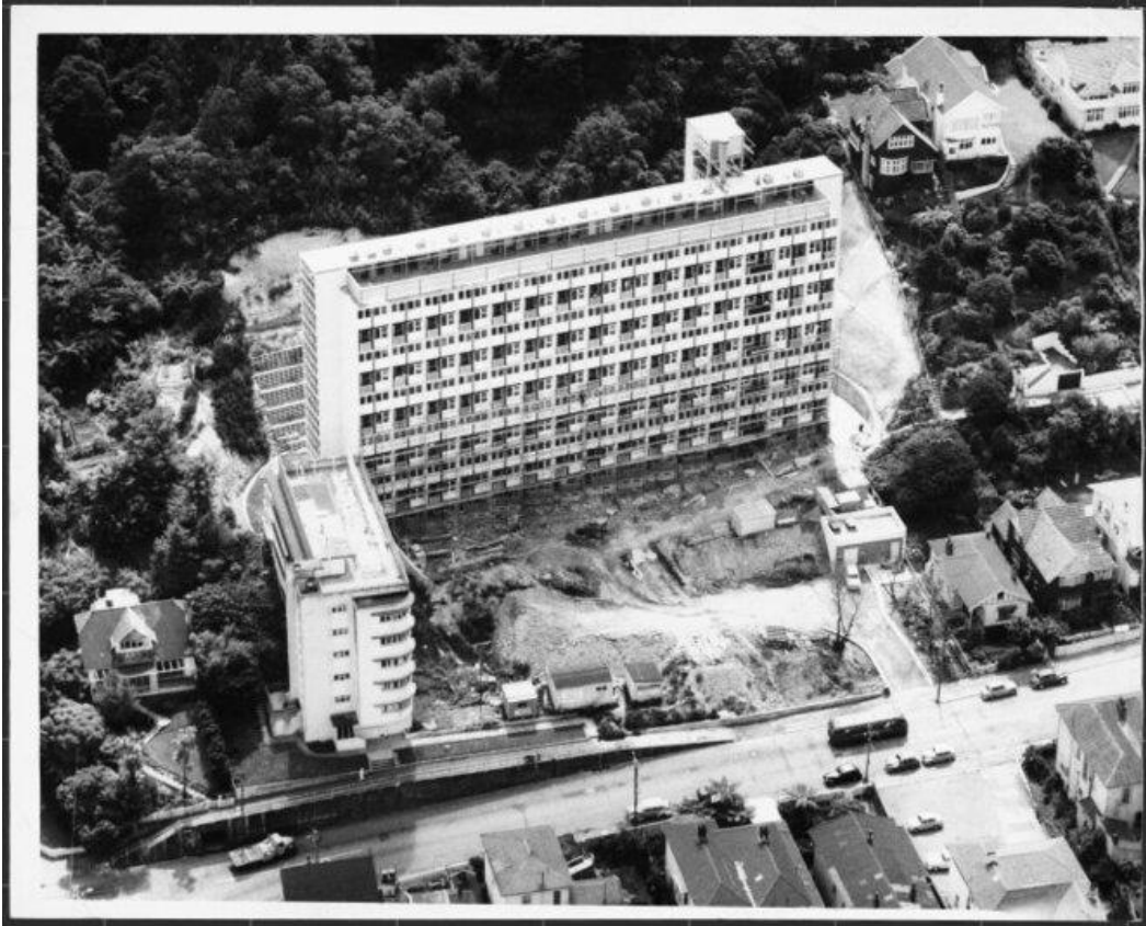
Figure 7: Gordon Wilson Flats under construction, 4 February 1958. EP-Industry-Housing-State-02, Alexander Turnbull Library, Wellington.
