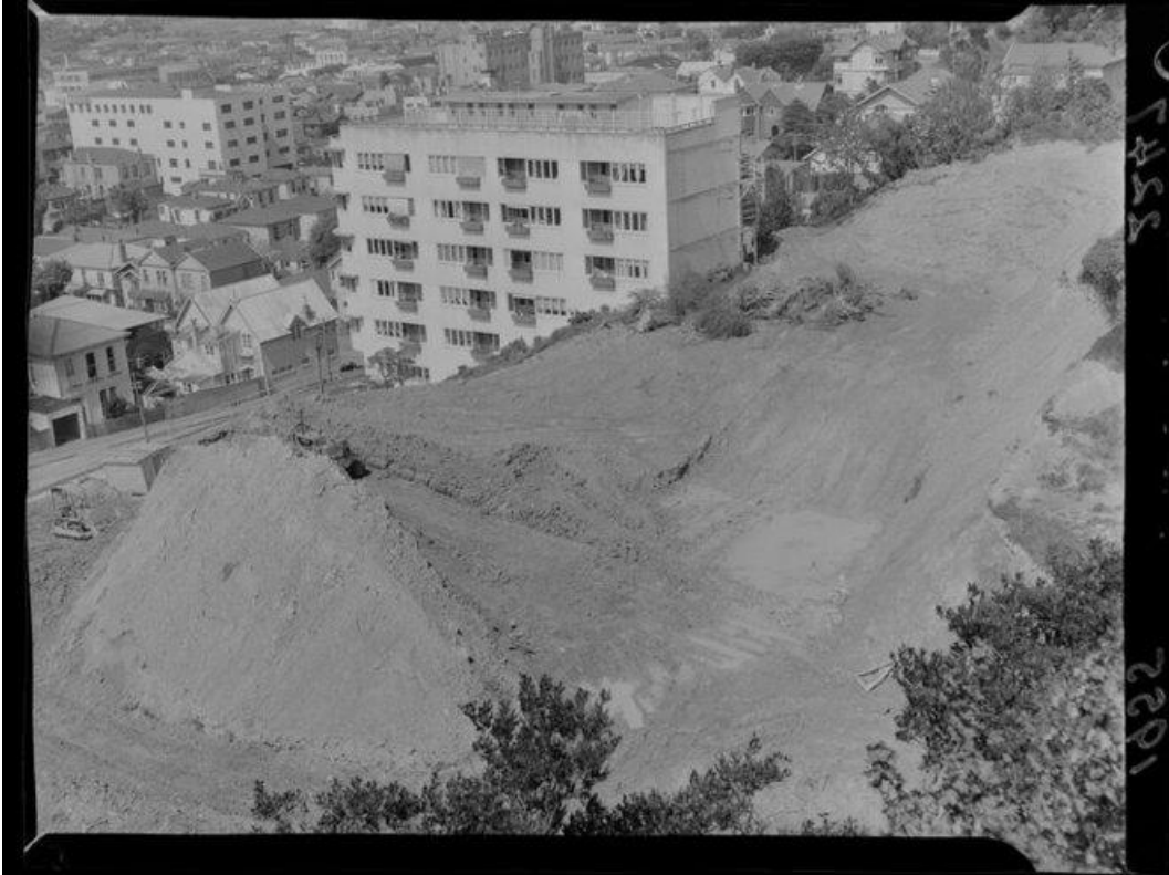
Figure 5: McLean Flats with earthworks for Gordon Wilson Flats, 1955. EP/1955/2247-F, Alexander Turnbull Library, Wellington. Note that the image shows the McLean Flats prior to the enclosure of their north-facing balconies.
