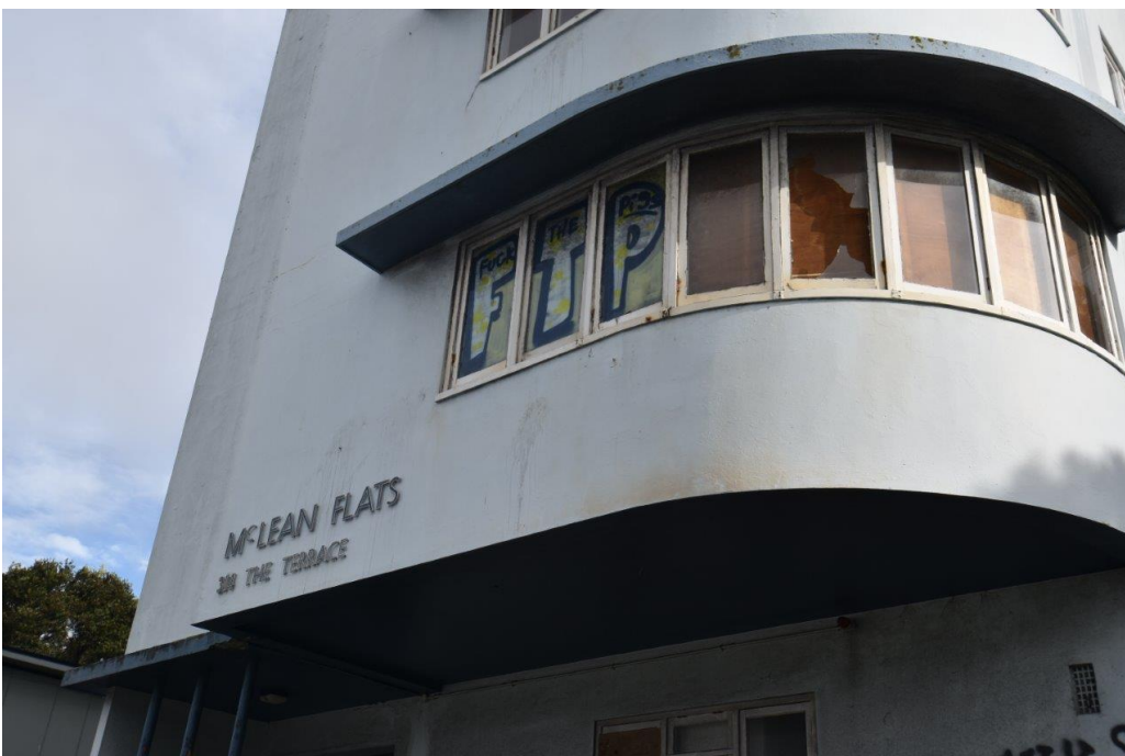
Figure 10: Detail of east elevation of McLean Flats.
