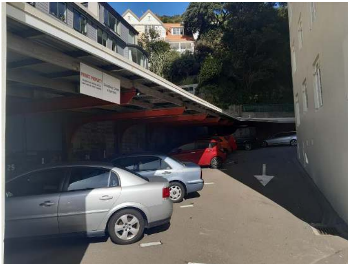
Figure 2: Photo of the carports on the eastern side of the property
