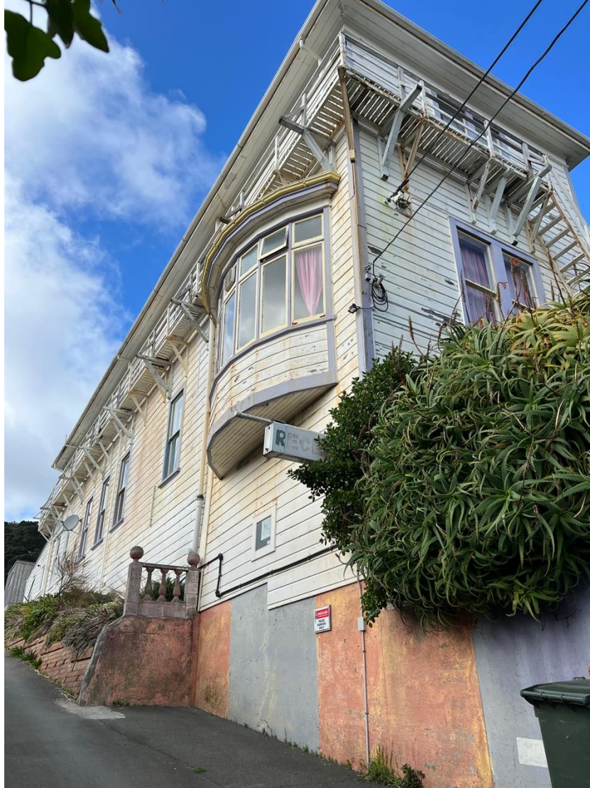
Figure 10 North west corner, 1 September 2022, Ian Bowman
