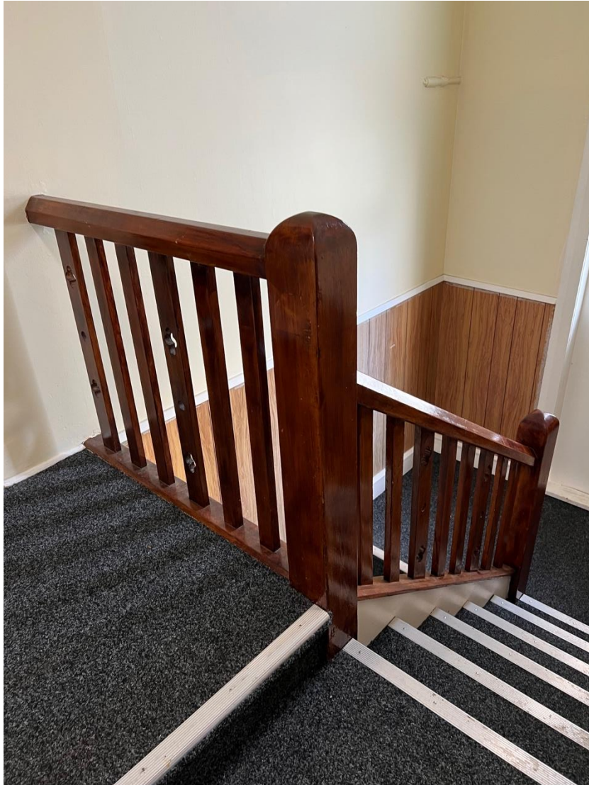
Figure 17 Stair, 1 September 2022, Ian Bowman
