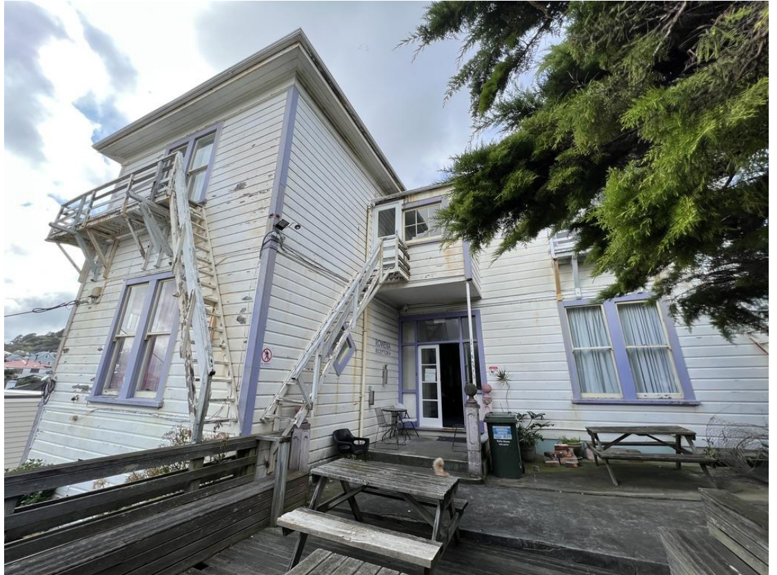
Figure 14 West elevation, 1 September 2022, Ian Bowman
