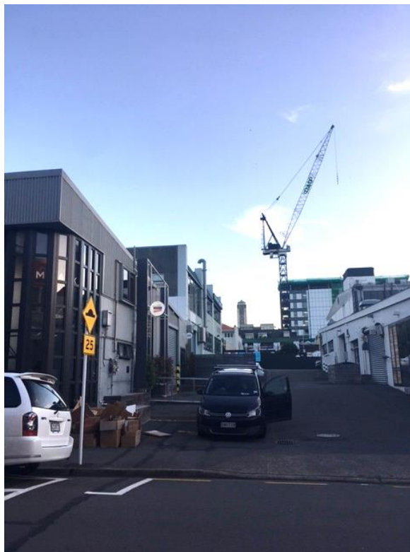
Fig 3: Photo from the footpath opposite service lane at 14 Jessie Street
