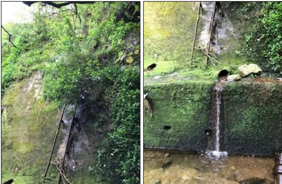
*An access ladder leans up the dam and pipes set into the dam help drain water (Daubé & Wellington City Council, 2022).*
