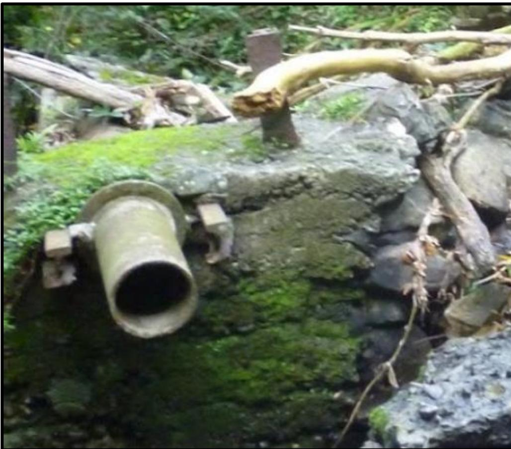
*View of stream. Note on far left of image is stonework covered in a layer of concrete. During the nineteenth century, stone dams were sometimes covered in a layer of concrete for protection (Cadenhead, 2023; Greater Wellington Regional Council, 2007).*
