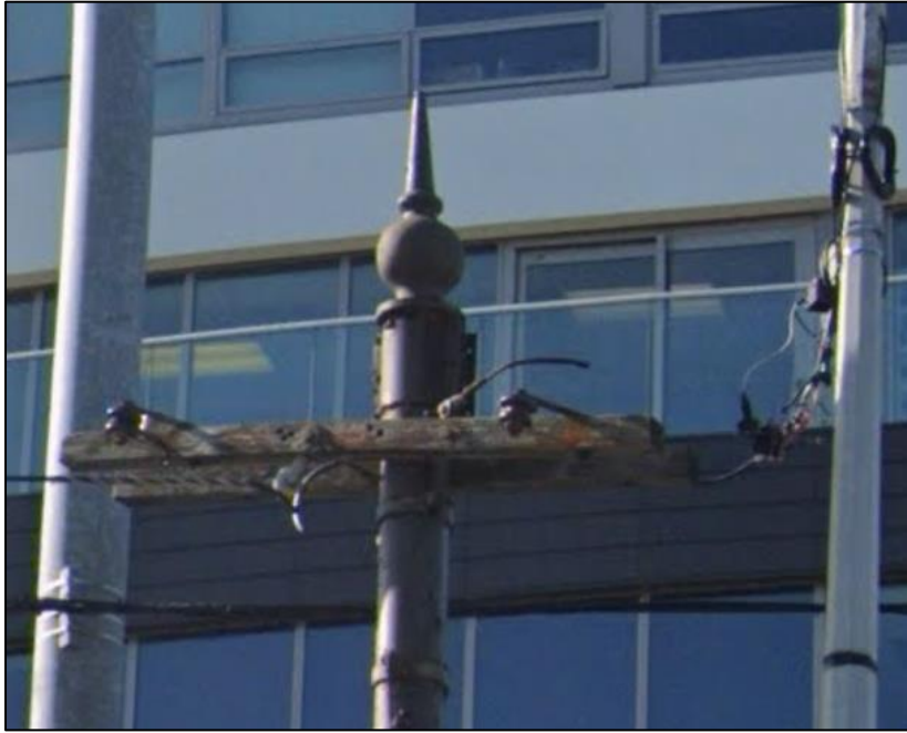
A close up view of the top of the Tram Pole as it stands today. Note insulators and wires (Google Street view September 2022).
