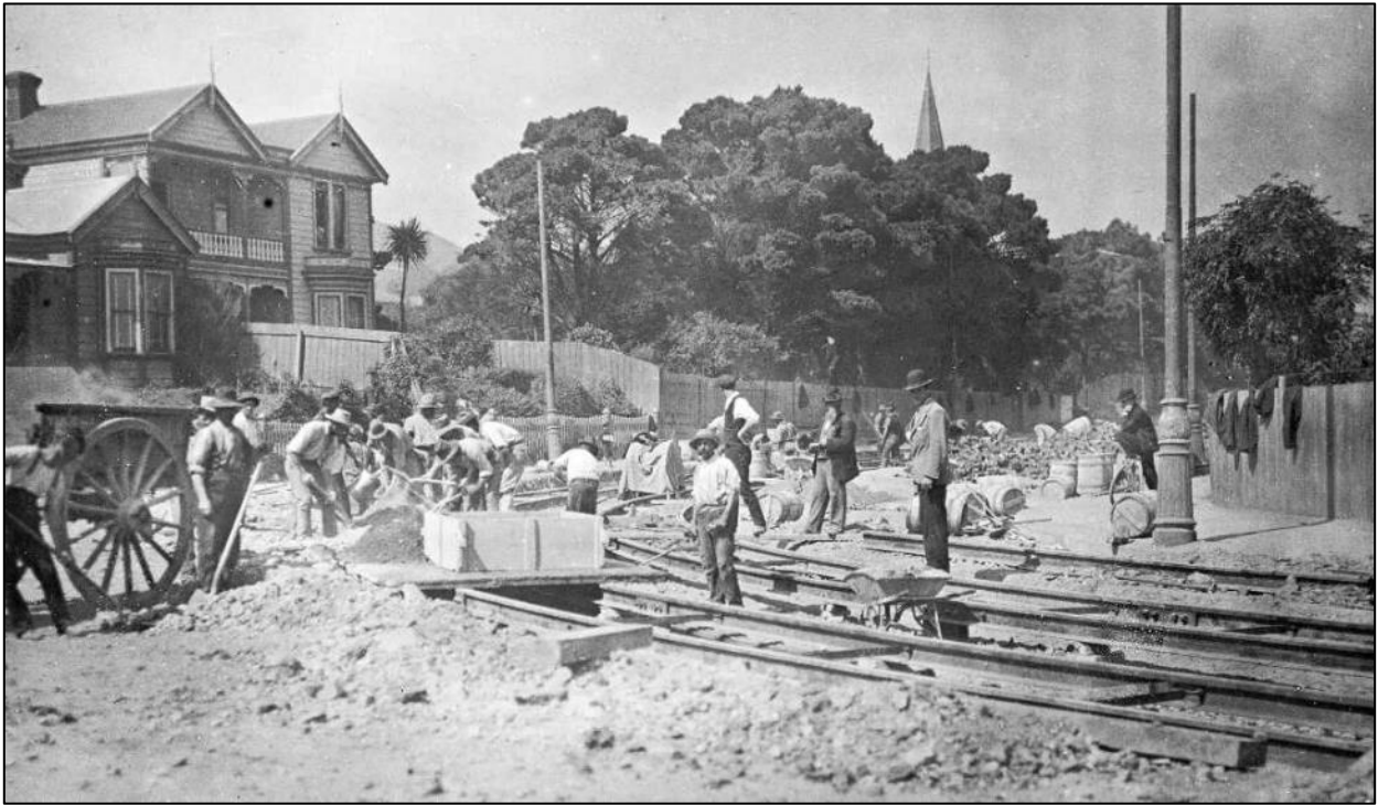
"Laying tram lines along the Basin Reserve, Wellington" (Unknown, 1900).
