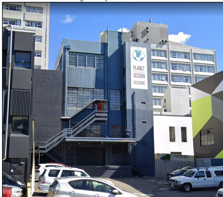
Rear of Building, 180 Victoria Street. Google Street View 2020.
