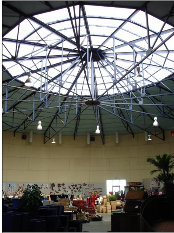
View of the glazed portions of the roof added in 1992. From Wellington City Council, "Gas Tank (Former) 139 Park Road PFG Summary Report.
