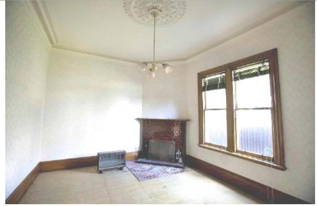
The dining room fireplace has been replaced with a timber surround and the dining room hatch has been moved to the north wall of the room.
