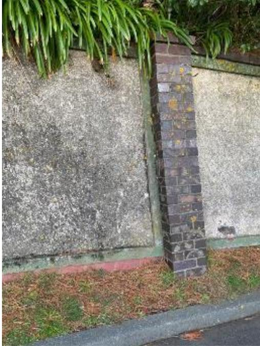
*Figure 6. Detail of eastern retaining wall at lower driveway showing brick pilasters, concrete infill, timber frame, and brick coping. Note non-original concrete kerb.*
