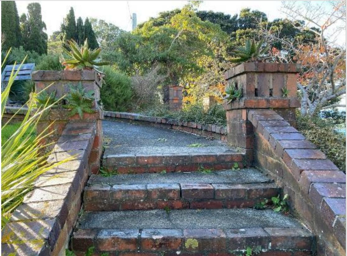
Figure 65. Piers at top of mausoleum entry steps. Note brick risers, brick walls. The group of four lower piers on the 'down loop' drive is visible in distance.
