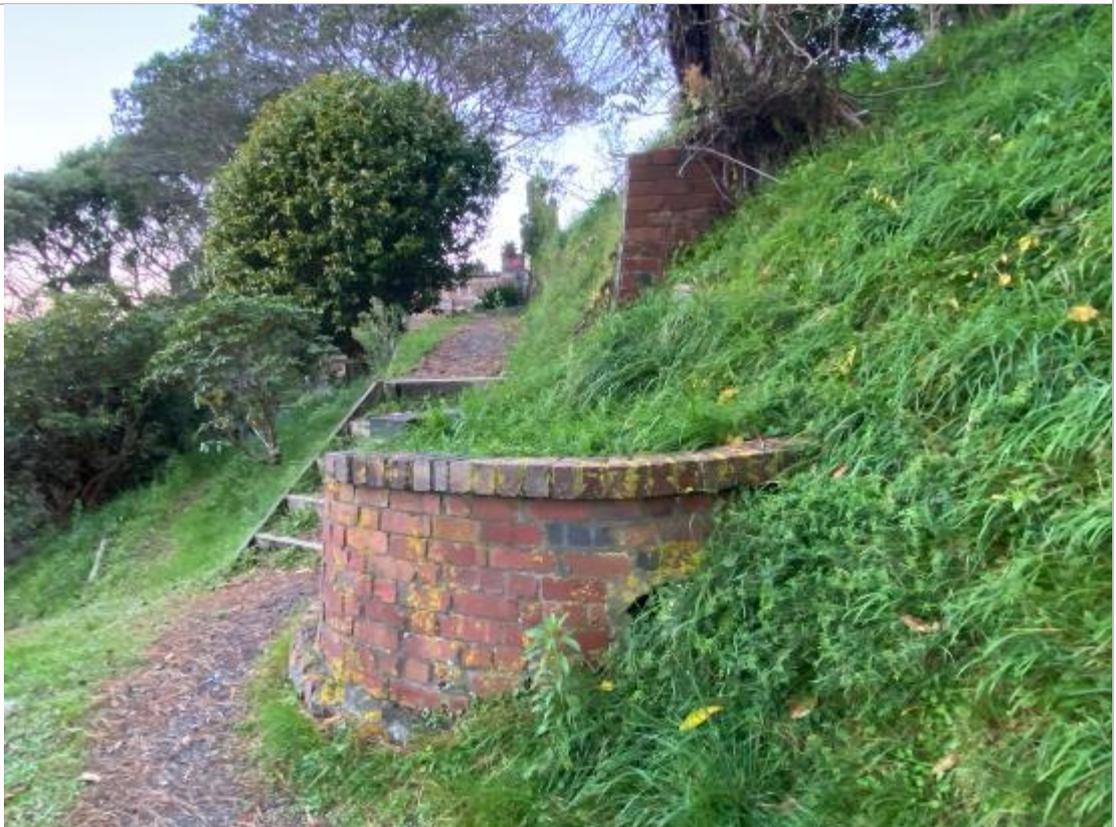
*Figure 52. A curved retaining wall/planter and pier a short way down the northern entry to dell.*
