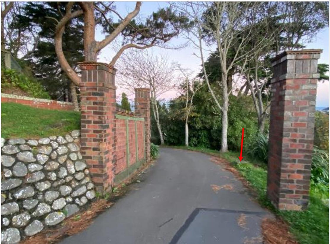
Figure 40. The upper group of three piers on the 'up loop' driveway, viewed from north. Note foundation for missing pier.
