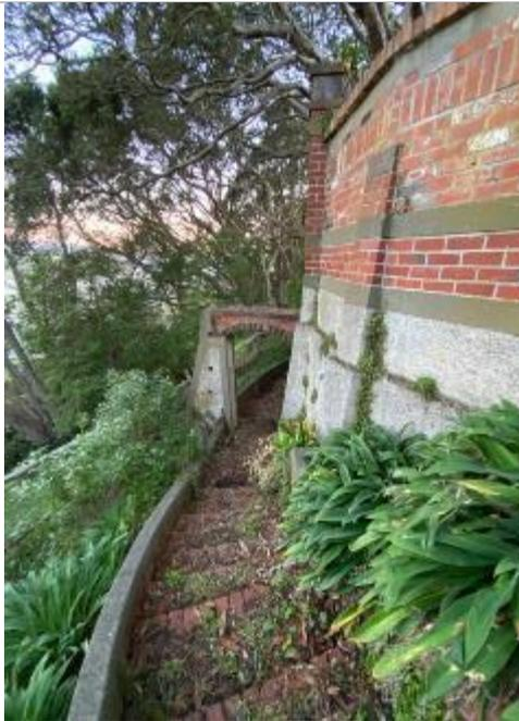
Figure 56. View from steps down behind semi-circular viewing platform. Note arch and contrasts between brick and concrete and plaster.
