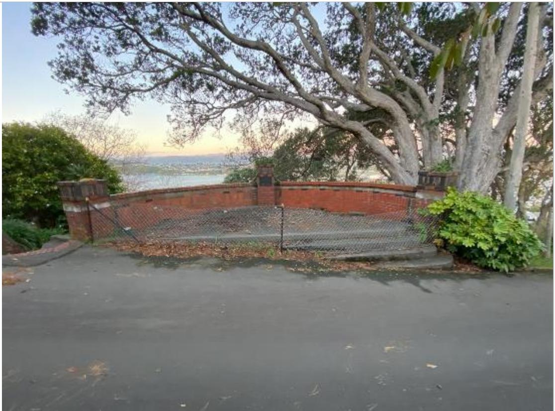
*Figure 54. Semicircular viewing platform and passing bay between the two groups of piers on the 'down loop' drive. Note integrated planters, and plaque.*
