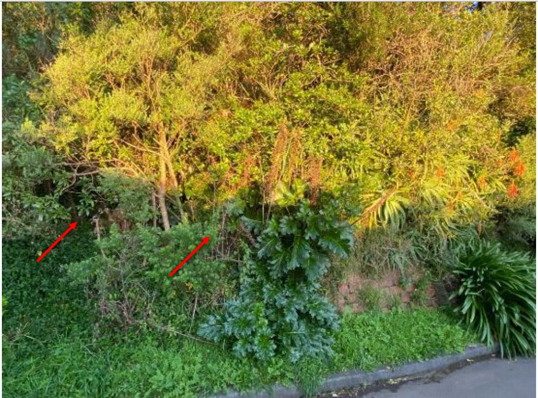
*Figure 7. This is a gap in the eastern retaining wall in the lower driveway. The land steps back and there are brick pilasters hidden in the undergrowth.*
