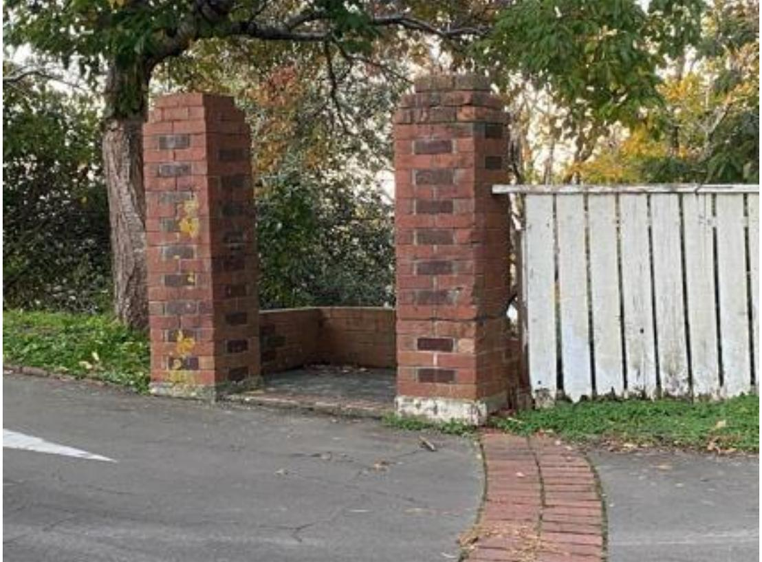
*Figure 28. This pair of columns mark the southern entry to the dell. Note top shaping that is different to that seen in retaining walls. Note brick 'threshold' in asphalt to mark the house grounds extent.*
