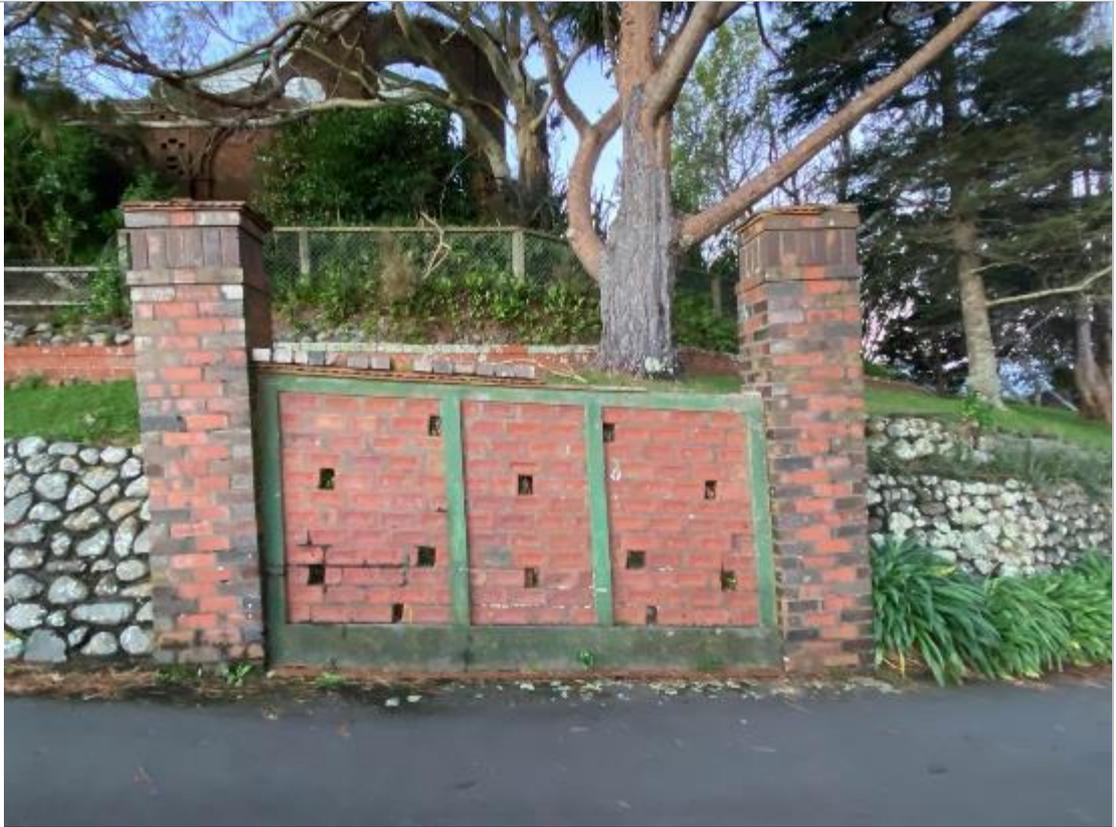
*Figure 41. The western retaining wall at the upper group of four piers on the 'up loop' driveway. Note random rock retaining walls to either side.*
