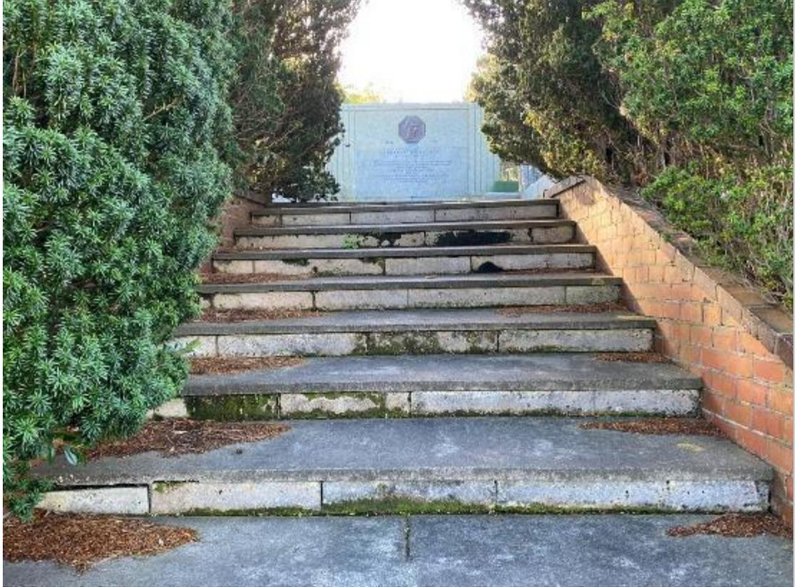
*Figure 69. Steps up to roof of mausoleum and plaque. Note that these stairs do not have brick risers – it appears to be a stone. Treads are concrete.*
