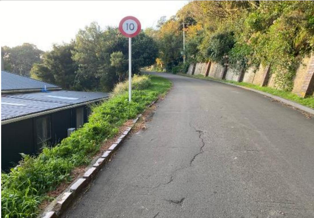
*Figure 4. View north up lower area of driveway. Note brick end-to-end kerb on west (LHS), and concrete kerb with brick/concrete retaining wall to east (RHS).*
