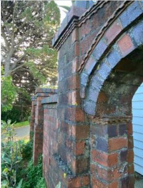
*Figure 74. Detail of brick wall at arch. Note terracotta tiles used to provide decorative edging, and also make up heights.*
