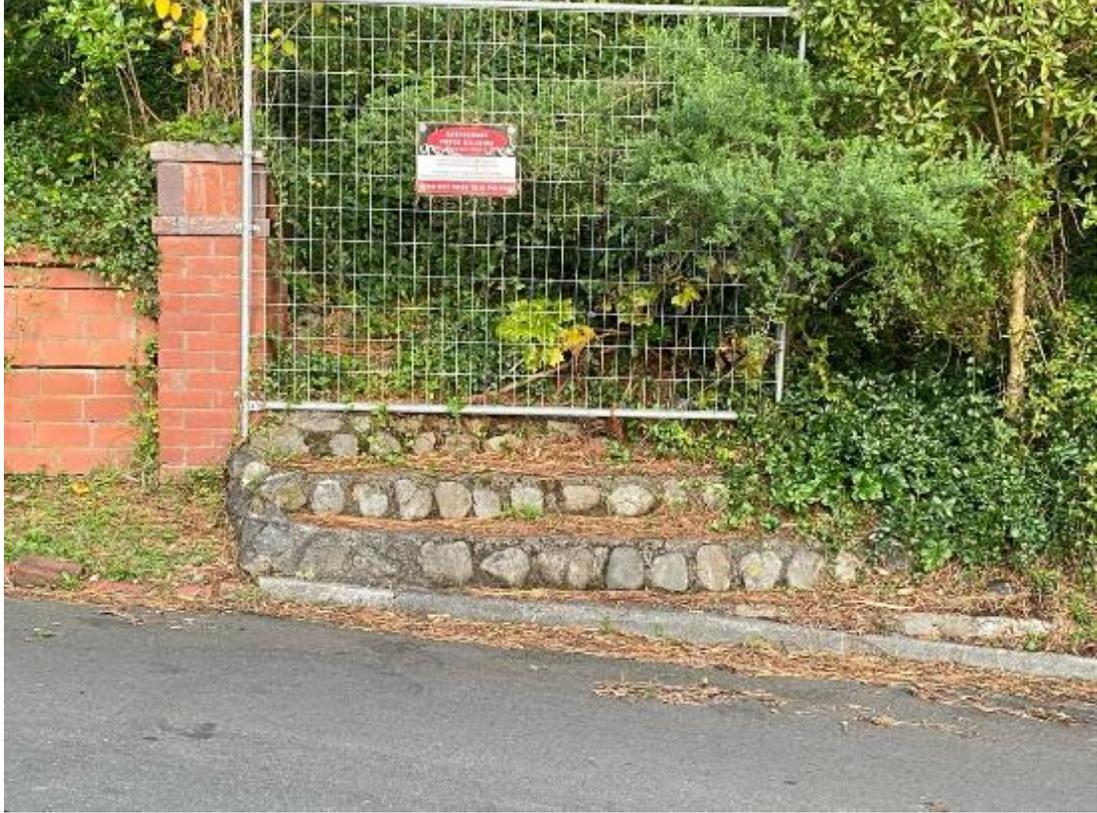
*Figure 15. 'Rock' steps to former site of hospital. Note no retaining wall to south (RHS). Brick kerb at north changes to concrete kerb.*
