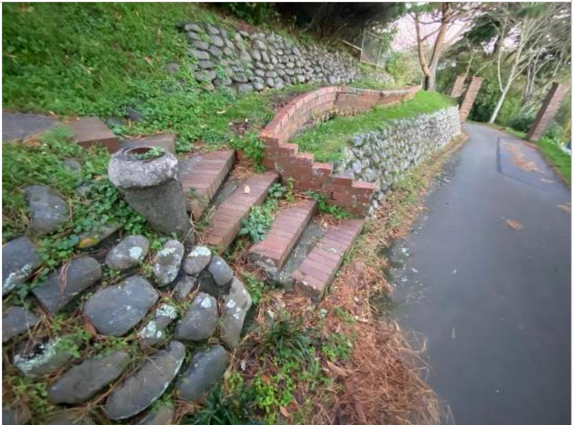
*Figure 42. Brick stairs and mid-level retaining wall towards the top of the 'up loop' driveway. The upper group of piers is in the distance.*
