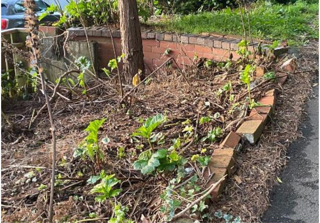
*Figure 14. Retaining wall at west of lower drive forming passing bay? Note difference in brick orientation on coping for retaining wall and kerbing.*
