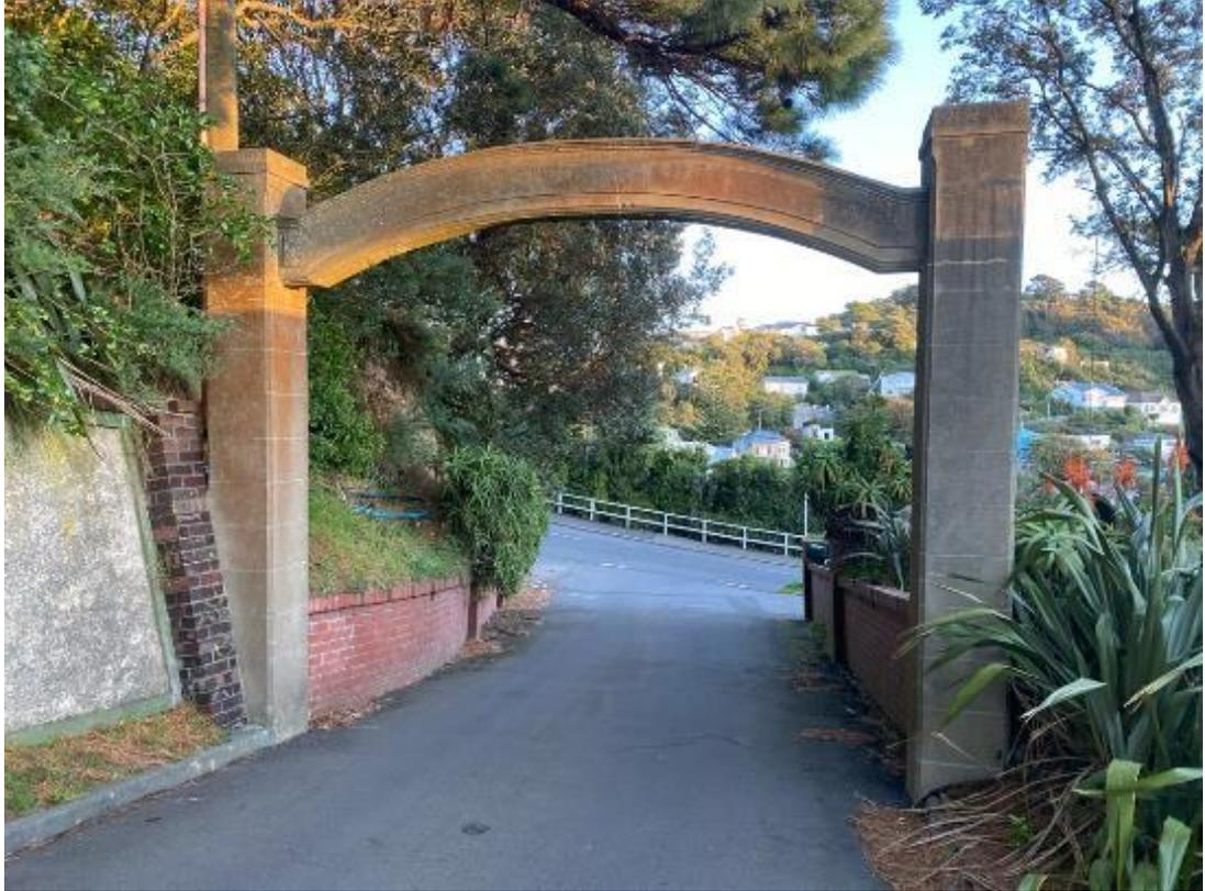
*Figure 3. Entry Arch 'Karitane' looking to Melrose Rd. Note fine detailing to plasterwork to give relief and imitation stone lines on columns.*
