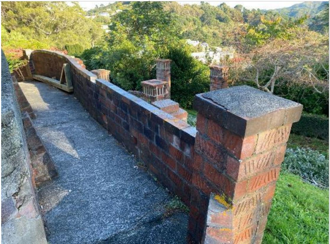
*Figure 68. Path around mausoleum at the west. Note diamond 'treads' inscribed in concrete, and figures in brick work.*
