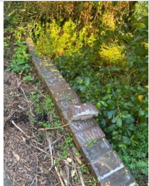
*Figure 13. Side-to-side bricks as a coping - possibly this is a retaining wall rather than a kerb. Note it changes to a kerb in the distance.*
