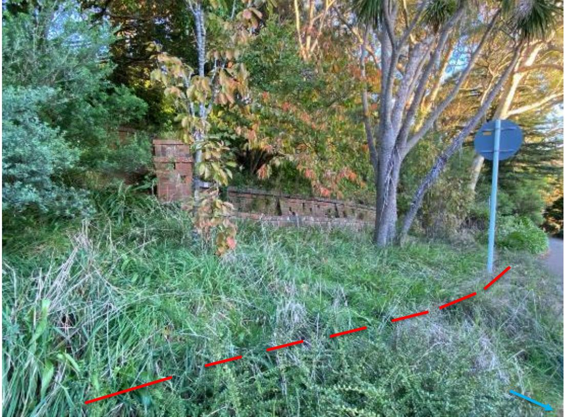
Figure 17. View of path from middle driveway. Pillar is at first zig-zag where path turns back to the south (to the right). Note that there is a low retaining wall (red) hidden under vegetation at bottom of picture, and a brick kerb below that (blue).
