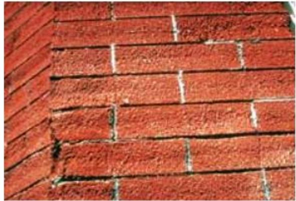
Sandblasting has permanently damaged this brick wall. Photo: NPS files
