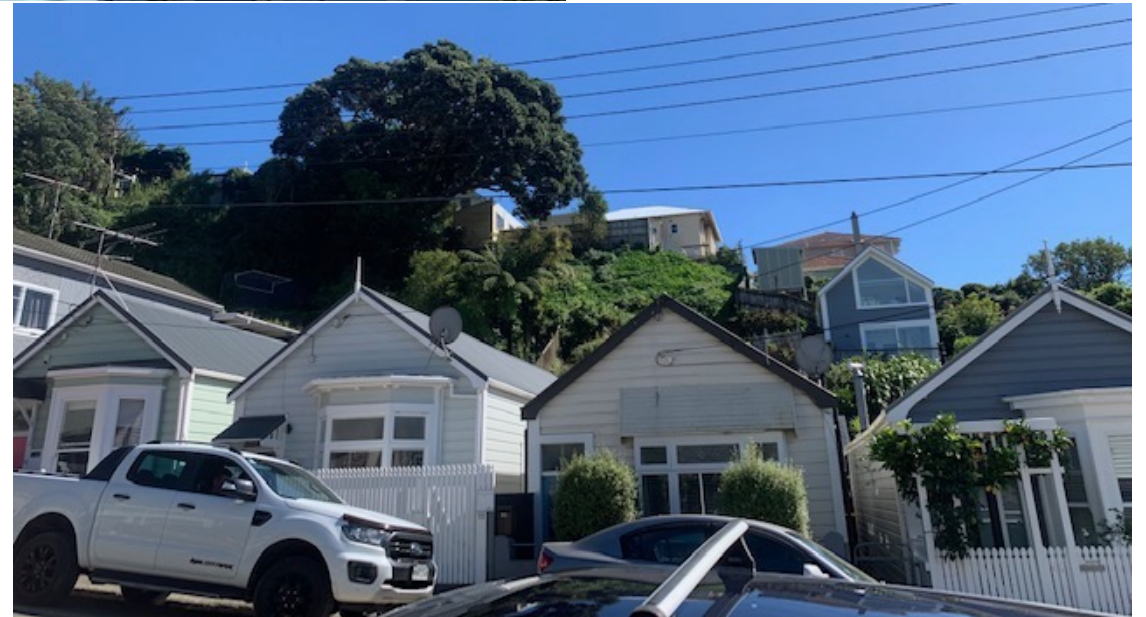
24 – 102 Rolleston Street, MOUNT COOK
