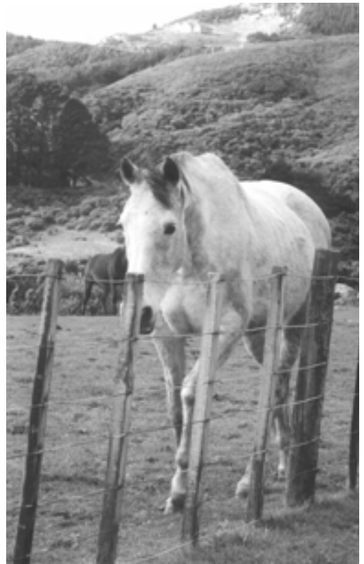
Typical rural 7-wire post and batten fence
