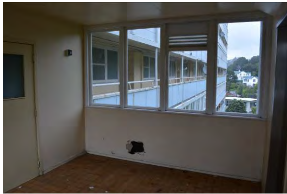
Figure 46. Looking at a typical lift lobby. (Archifact-Architecture & Conservation Ltd., 2014)
