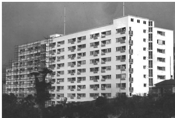
Figure 73. Dixon Flats nearing completion in 1944. (Source: Gatley, J, 2008, page 42)
