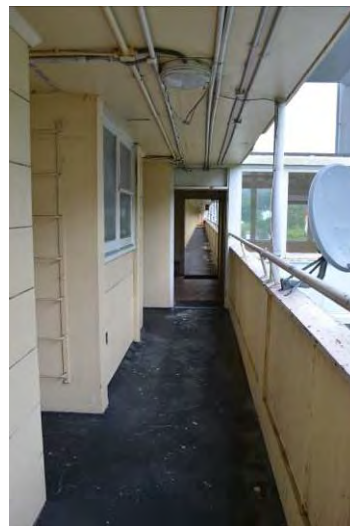
Figure 44. Looking south along a typical walkway. (Archifact-Architecture & Conservation Ltd., 2014)
