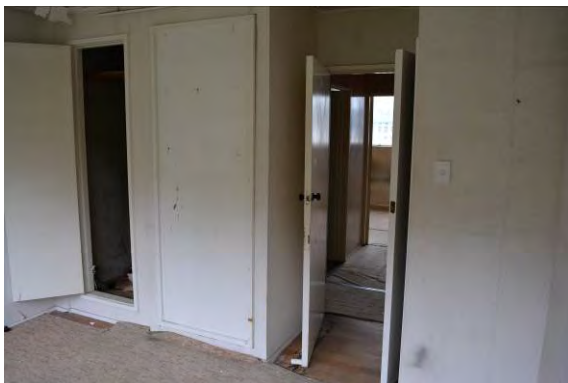
Figure 59. Looking at a typical west side bedroom. (Archifact-Architecture & Conservation Ltd., 2014)
