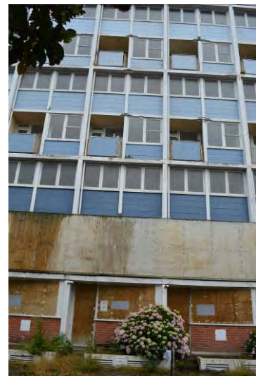
Figure 26. Looking at the lower levels of the eastern elevation. Note the Ground Floor level apartments are boarded over preventing access into the interior. (Archifact-Architecture & Conservation Ltd., 2014)
