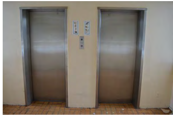
Figure 47. Looking at a typical set of lift doors. (Archifact-Architecture & Conservation Ltd., 2014)
