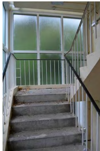
Figure 41. Looking at a typical stairwell positioned at the north and south ends of the building. (Archifact-Architecture & Conservation Ltd., 2014)
