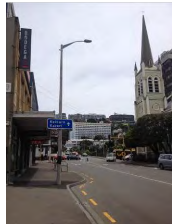
Figure 15. Looking north-west towards the Gordon Wilson building from the junction of Victoria Street with Ghuznee Street. (Archifact-Architecture & Conservation Ltd., 2014).
