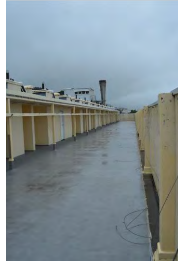
Figure 29. Looking south along the open roof deck. Note the laundry and storage rooms to the left of the image. Also note the flue serving the buildings boiler house. (Archifact-Architecture & Conservation Ltd., 2014)
