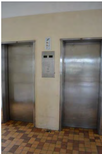
Figure 40. Looking at the main passenger lift entrance lobby at Ground Floor level. (Archifact-Architecture & Conservation Ltd., 2014)
