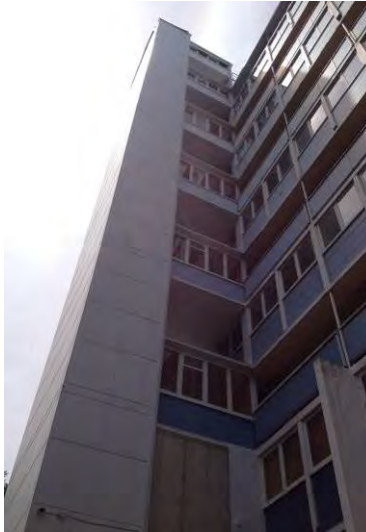
Figure 21. Looking north at the lift tower and its junction with the west elevation. (Archifact-Architecture & Conservation Ltd., 2014)
