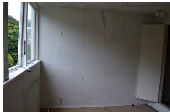
Figure 60. Looking at a typical west side bedroom. (Archifact-Architecture & Conservation Ltd., 2014)
