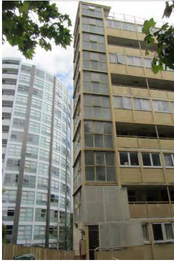
Figure 91. Stairwell to north side of flats. (Archifact-Architecture & Conservation Ltd., 2014)
