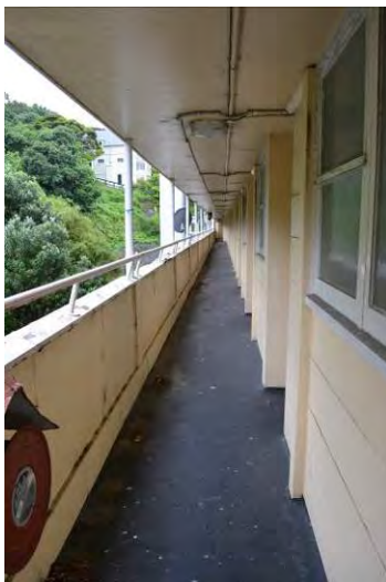
Figure 43. Looking north along a typical balcony walkway providing access to flats. (Archifact-Architecture & Conservation Ltd., 2014)
