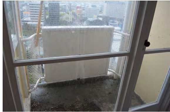
Figure 55. Looking out towards a typical balcony that serves each of the flats. (Archifact-Architecture & Conservation Ltd., 2014)
