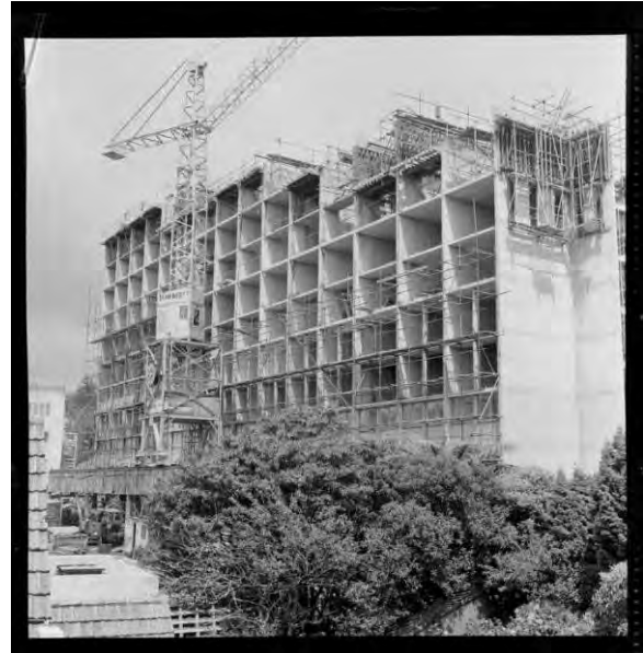
Figure 7. Terrace flats under construction, The Terrace, Wellington. Negatives of the Evening Post newspaper. Ref: EP/1957/4364-1-F. Alexander Turnbull Library, Wellington, New Zealand. http://natlib.govt.nz/records/23246983
