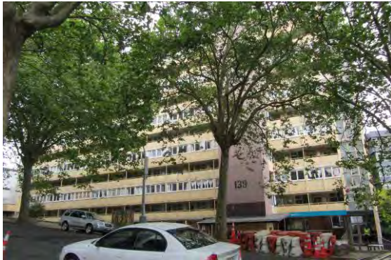
Figure 87. Street view of flats, partially obscured by mature trees at the street side. (Archifact-Architecture & Conservation Ltd., 2014)
