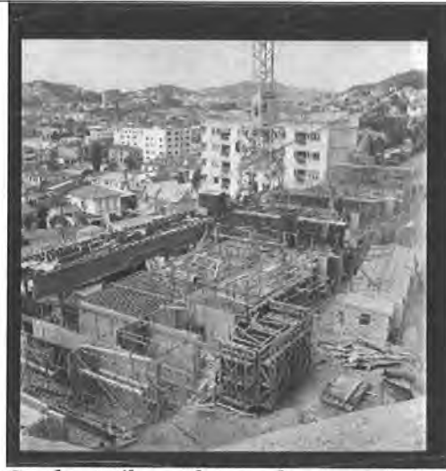
Gordon Wilson Flats under construction circa 11 February 1957. The McLean State Flats are behind the Downer crane. Evening Post . (Timeframes EP/1957/0397-F)
