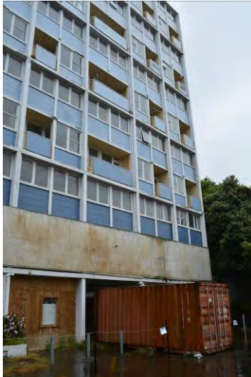
Figure 27. Looking at the northern end of the eastern elevation. Note the steel shipping container slotted into the main entrance to protect visitors from falling debris. (Archifact-Architecture & Conservation Ltd., 2014)
