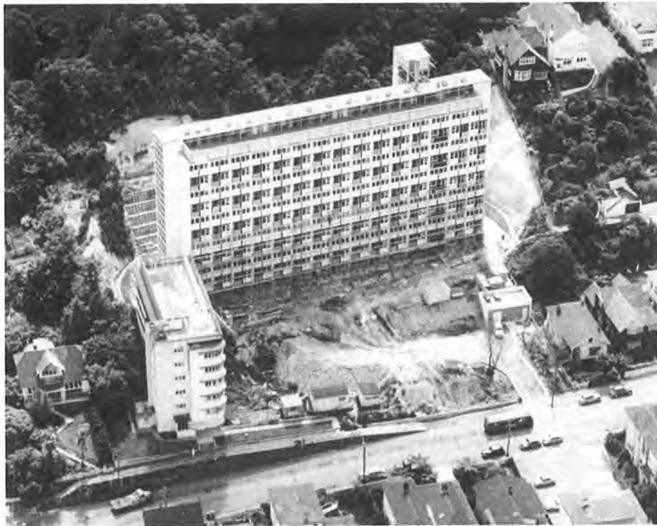
Aerial view of the Gordon Wilson Flats under construction c1958-9. The McLean State Flats are to the left (Ref: EP-Industry-Housing-State-02, ATL)
