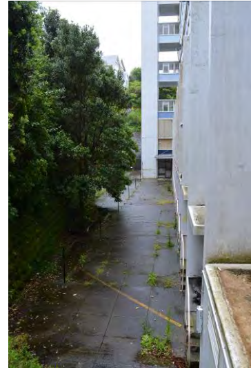
Figure 23. Looking north along the western elevation. Note the slender buttresses on the right of the image that act as stiffening members anchoring the structure to the pile heads. (Archifact-Architecture & Conservation Ltd., 2014)
