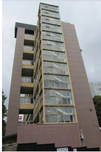
Figure 92. Stairwell to south side of flats. (Archifact-Architecture & Conservation Ltd., 2014)
