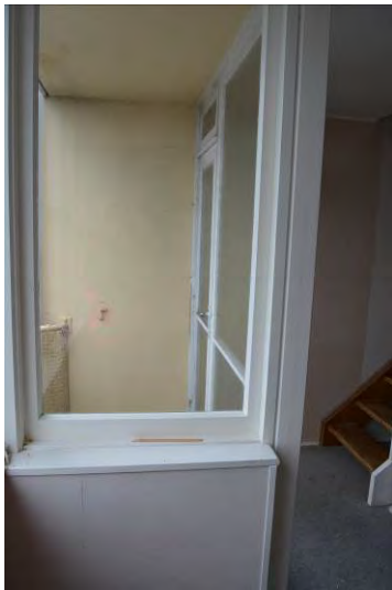
Figure 54. Looking at a typical balcony enclosure. (Archifact-Architecture & Conservation Ltd., 2014)
