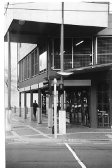
Building frontage to the street
