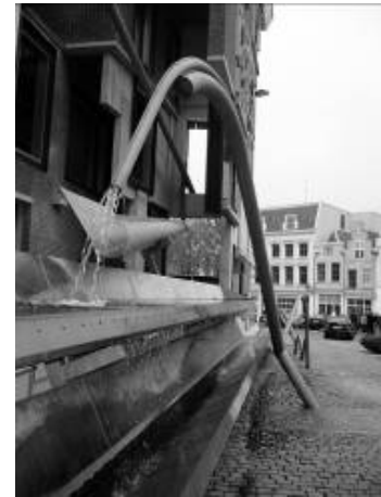
Richness of detail at ground level
