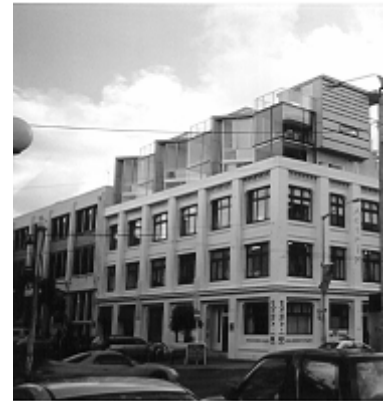
Example of relating to context with vertical alignment and completion of the composition of an existing building with a new top
