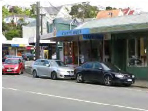
Narrow, single storey frontages to the north side of Upland Road
