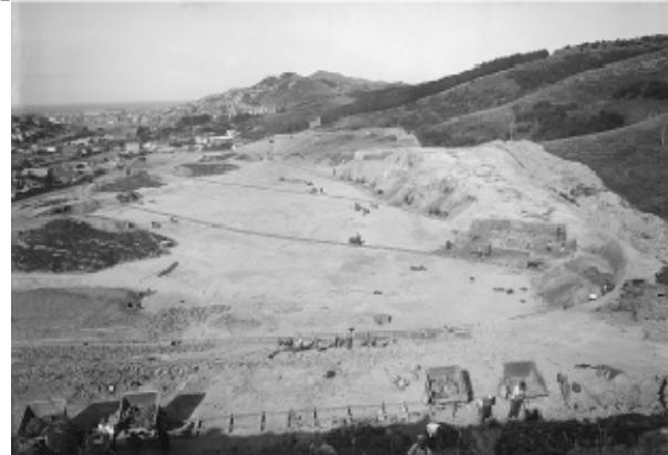
**Figure 4: Hataitai Park under construction in 1932. Relief labour dug out banks and moved spoil in metal bins on rails. Spoil from the Mount Victoria tunnel was also used to form the park.**
