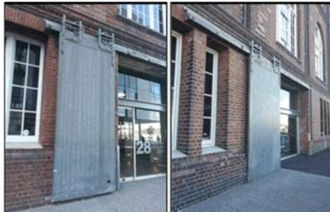
Figure 4. Left: historic door and track system. Right: replica door and track system.
