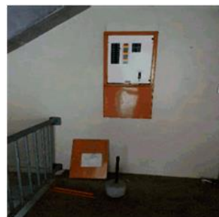
Figure 231: Distribution board with cover removed
