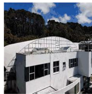
Figure 27: Various cladding materials to the north end of the main building
