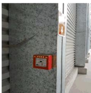
Figure 108: Manual Call Point
