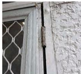
Figure 159: Rusty hinge
