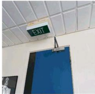
Figure 92: Incorrect mount for illuminated 'Exit' sign. The word 'exit' should be in a vertical position.
