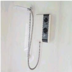
Figure 143: Electric continuous flow shower unit.
