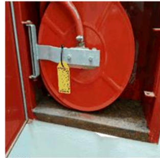
Figure 93: Expired Fire Hose Reel
