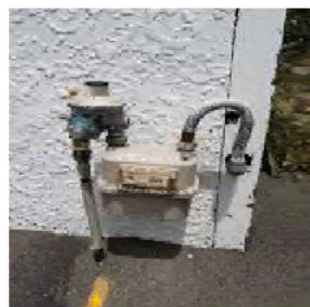
Figure 183: Uncovered gas meter adjacent to public foot path
