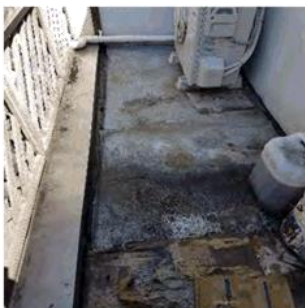
Figure 22: Damage to deck area caused by user chemicals
