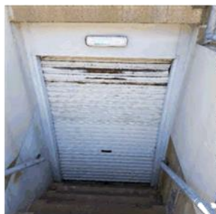
Figure 210: Failed roller door from the stand area into the concourse
