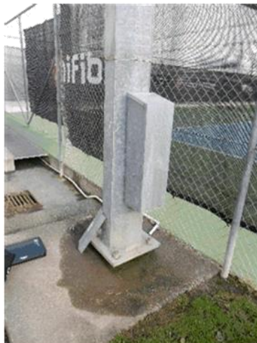
Photo – Outdoor courts typical pole internal condition (left) and floodlight gear tray enclosures on pole base
