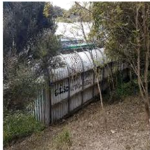
Figure 240: Colorsteel cladding to stand
