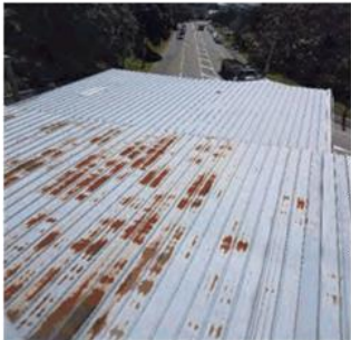
Figure 150: Metal roof showing extensive rust
