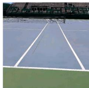
Figure 112: Cracking to court surface
