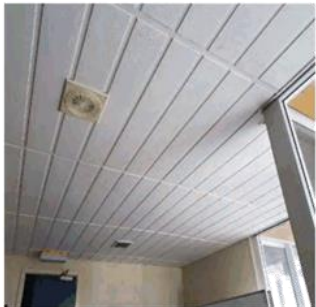
Figure 53: Heavy plaster ceiling tile to the first floor
