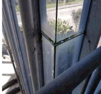
Figure 9: Movement in the glazing panels around the stairwell
