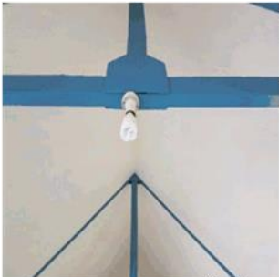
Figure 142: Single Bayonet light fitting
