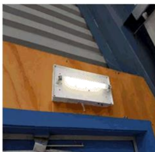
Figure 3: Illuminated exit sign cover is broken and no longer displays the word 'Exit'
