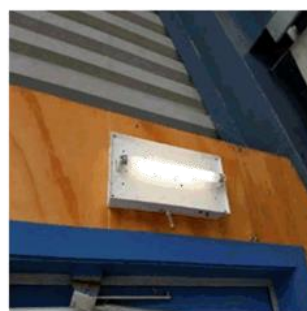
Figure 109: Illuminated 'exit' sign with missing cover plate
