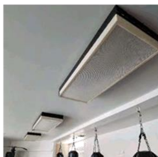
Figure 171: Fluorescence light fitting with defuses
