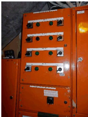
Photo – Indoor Courts 1, 2, 3 & 4 Lighting Control Panel
