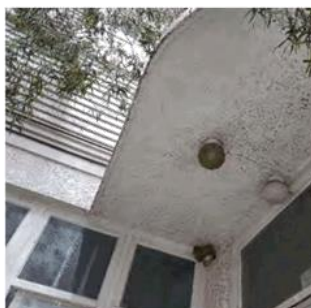
Figure 160: Light fittings to front door with fire siren in top corner
