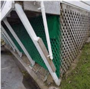
Figure 132: Downpipe discharges to the ground
