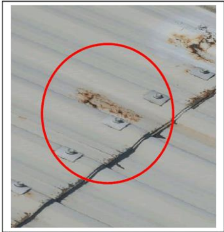
Corroding lap seam
