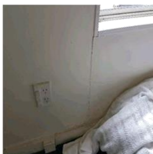
Figure 139: Crack to plasterboard join
