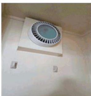
Figure 187: Extract system to shower area
