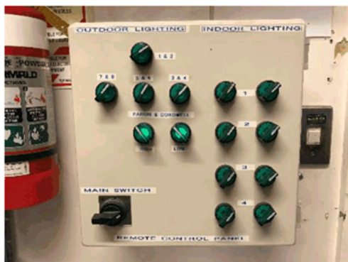
Photo – Court Lighting Remote Control Panel
