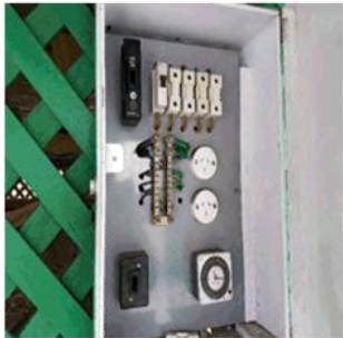
Figure 141: Distribution Board
