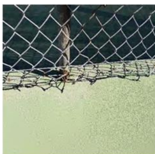
Figure 120: Corrosion to fence post
