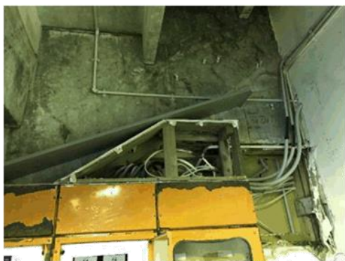
Photo – Submain and subcircuit cables into top of MSB1
