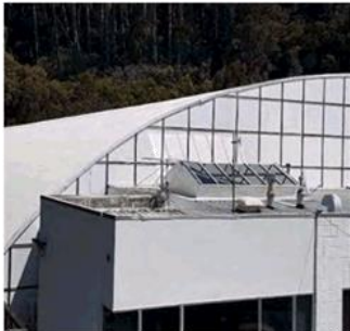
Figure 16: Penetrations to Administration roof
