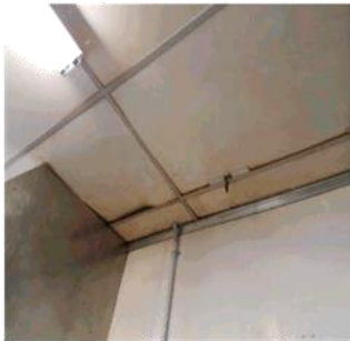
Figure 55: Ceiling tile to kitchen heavily stained
