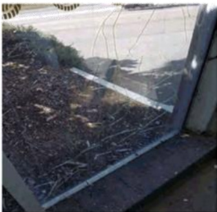
Figure 208: Cracked window pane
