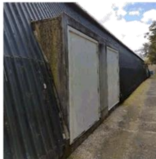
Figure 24: Egress doors to eastern side of the building should be check for cladding material
