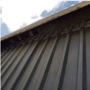
Figure 15: Oxidation occurring to top of roofing iron and netting failed
