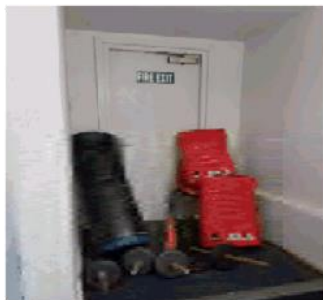
Figure 5: The gymnasium fire exit is blocked with equipment
