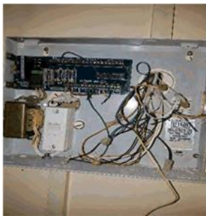
Figure 184: Internal wiring to security panel
