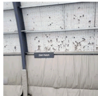
Figure 106: Damaged building paper.
