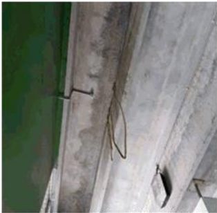
Figure 222: Corking hanging from ceiling
