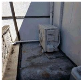
Figure 84: External unit to 1 st floor heat pump
