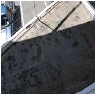
Figure 19: Failed deck off boardroom. To be checked for Asbestos content
