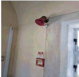
Figure 237: Manual call point and sounder
