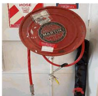
Figure 196: Fire hose drum in poor condition
