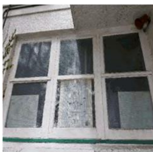
Figure 157: Painted timber framed windows
