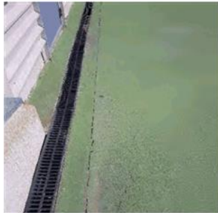
Figure 114: Cracking along surface drain
