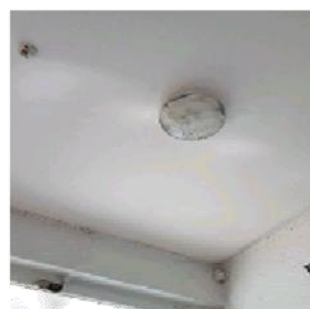
Figure 172: Surface mounted light fitting
