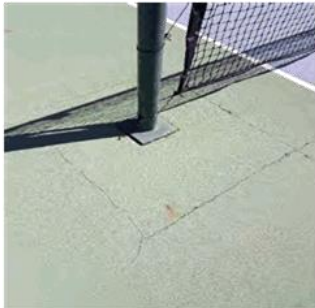
Figure 115: Cracking around netting support
