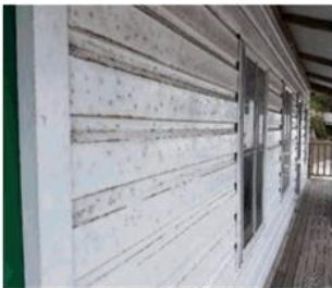
Figure 133: Cladding showing oxidation
