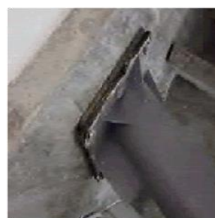
Figure 200: Close up of corroding internal steel bracing
