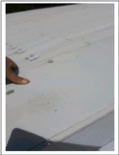
Lifting flashings
