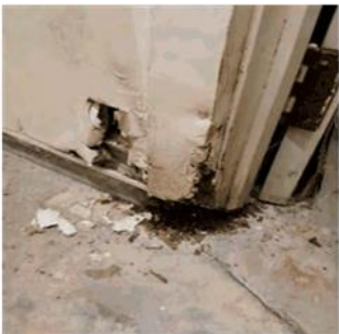
Figure 220: Damage to trims and linings are a result of water ingress
