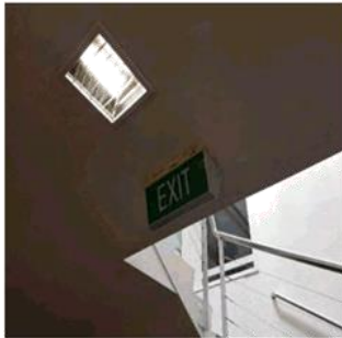
Figure 91: Illuminated 'Exit' sign but needs review as indicate exist up the stairs and not the nearest exit
