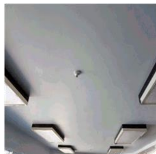
Figure 195: Heat detector
