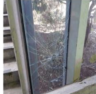
Figure 10: An example of the numerous cracked glazing panes to the North Stand
