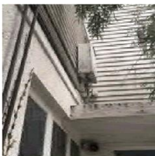
Figure 182: Instantaneous gas heating unit
