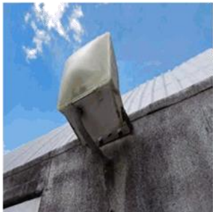
Figure 35: Rusting to light housing and bracket and UV damage to the fitting cover
