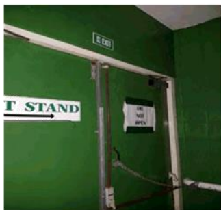
Figure 7: The North Stand fire exit door is chained shut and would not function as designed in the event of a fire
