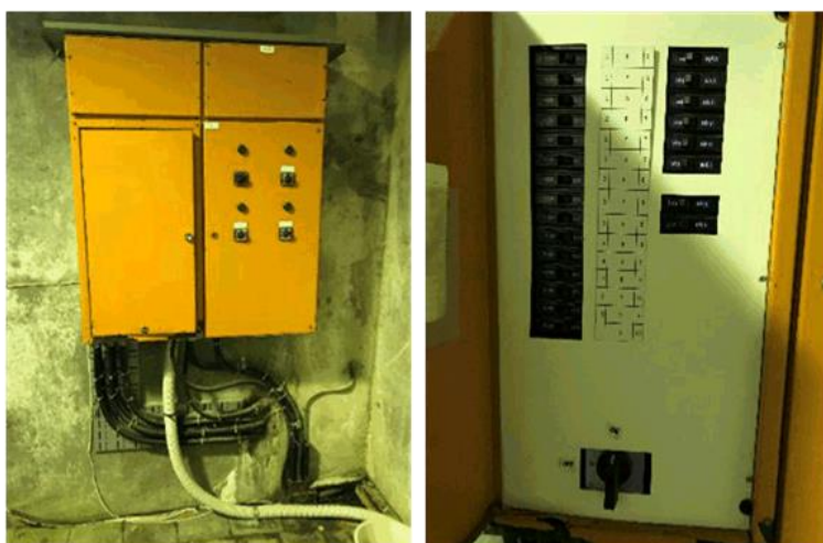
Photo – Outdoor courts lighting distribution board
