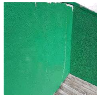
Figure 248: Cracking and failure of cladding
