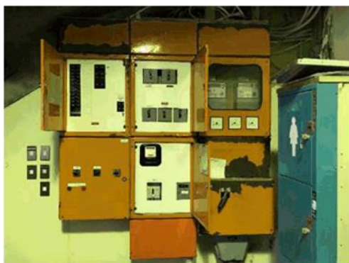
Photo – Main switchboard, North Stand, MSB1
