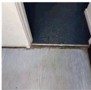
Figure 47: Vinyl to the first floor has been poorly laid
