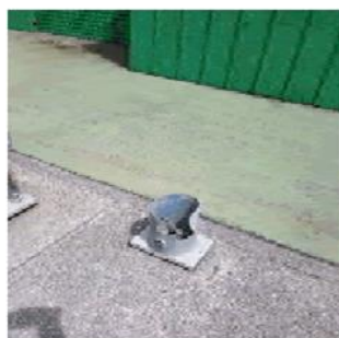
Figure 275: Hose tap protected by metal surround
