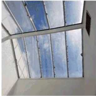
Figure 17: Skylight to lounge area showing moss and lichen to glazing
