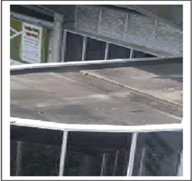
Pooling water in middle membrane roof
