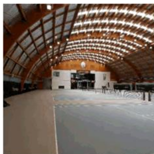
Figure 11: Exposed laminated wooden beams and purlins to court area
