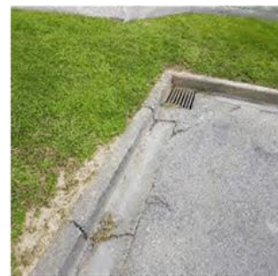
Figure 261: Failed concrete kerb and channel
