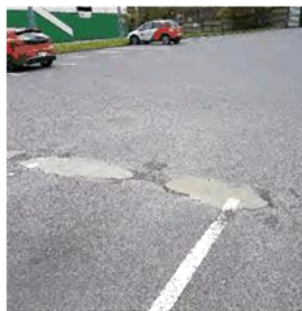
Figure 260: Pot whole requires further work to prevent substrate damage
