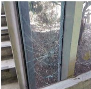
Figure 207: Cracked window pane
