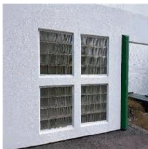
Figure 30: Glass bricks install to the ground floor changing room
