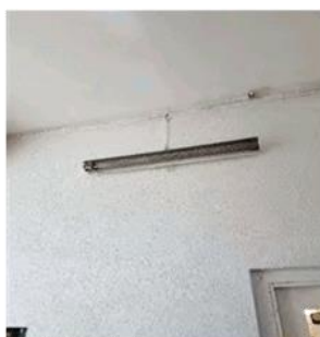
Figure 188: Bar heating to areas within the building
