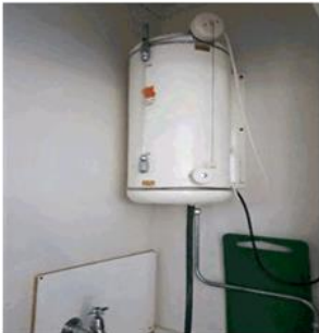
Figure 177: Zip boiler unit
