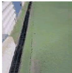
Figure 270: Crack that effects the sites drainage
