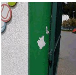
Figure 257: Failed paint system to steel posts
