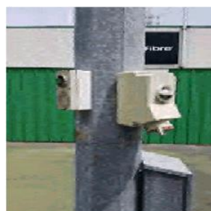
Figure 276: External power fittings to flood light pole
