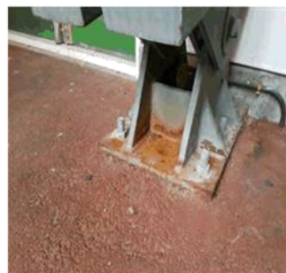
Figure 13: Early signs of rusting that should be remediated to prevent further corrosion
