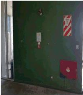
Figure 236: Fire Hose cabinet manual call point and sounder
