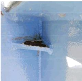
Figure 96: Steel lug that is corroding due to water pooling
