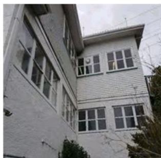
Figure 154: Cladding is a mix of plaster & weatherboard
