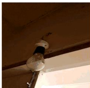
Figure 173: Bayonet fitting not securely
