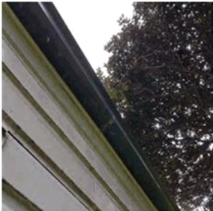
Figure 131: Example of spouting showing early signs of failure at the joins
