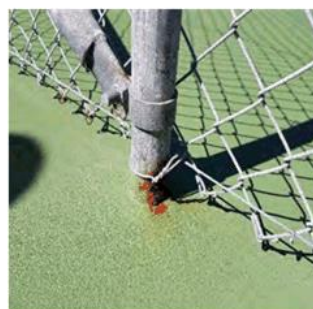
Figure 121: Corrosion to fence post
