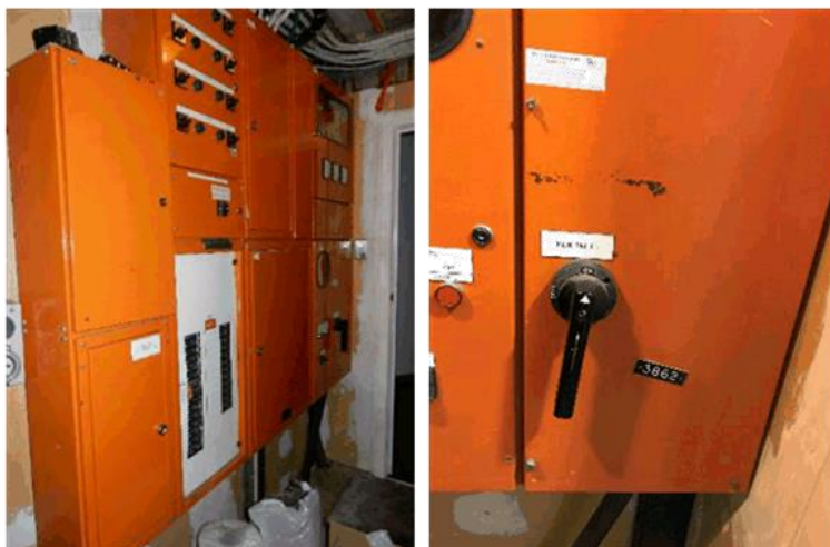
Photo – MSB2 and close up of main switch
