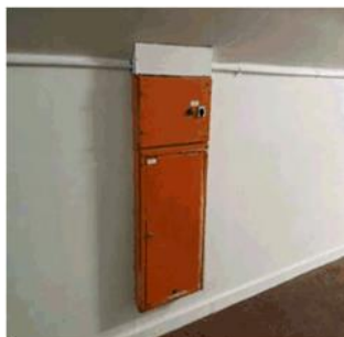
Figure 64: Distribution board to hallway area under gallery seating
