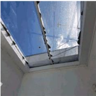
Figure 18: Skylight to top of eastern stairs showing moss and lichen to glazing
