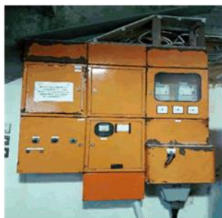
Figure 229: Switchboard housing in Very poor condition
