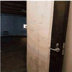
Figure 226: Failed paint system to internal door
