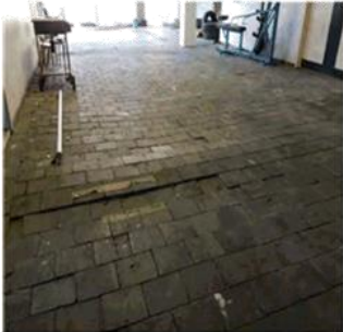
Figure 216: Concrete pavers present as a hazard
