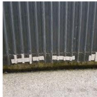
Figure 25: Aluminium tape covering failed sheet cladding
