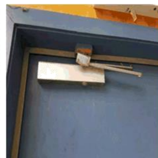
Figure 102: Failed door closer
