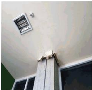
Figure 219: Failed ceiling due to water
