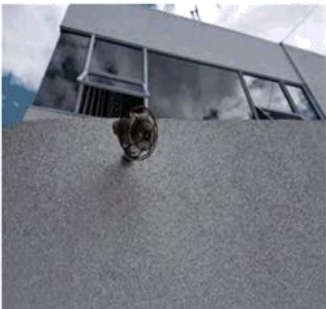
Figure 36: Rust to the metal protection cage
