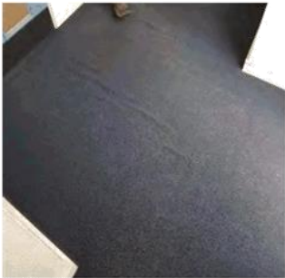
Figure 44: Carpet to level 1 offices needs to be re-stretched but also a lot of wear
