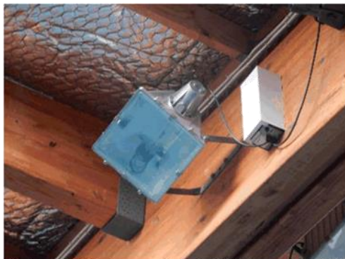
Photo – Main indoor courts typical Philips metal halide floodlight and adjacent control gear box
