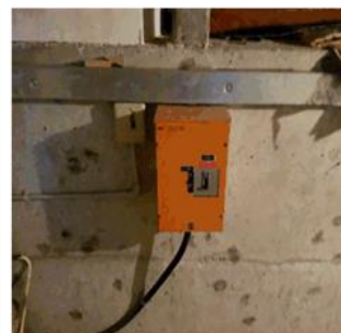
Figure 235: Power distribution box to the lift
