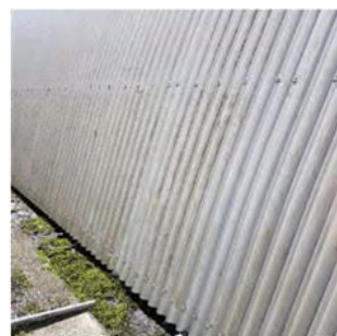
Figure 99: South side of building with foreign material and growth in the drainage system
