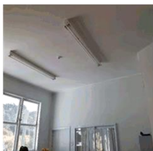
Figure 170: Fluorescence light fitting to office area
