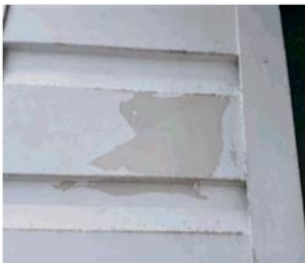
Figure 134: Paint membrane failure
