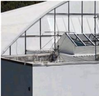
Figure 42: Aerial to roof with wire bundled around the stand
