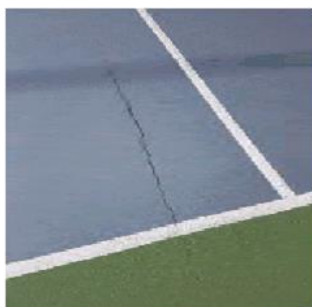
Figure 110: Cracking to court surface
