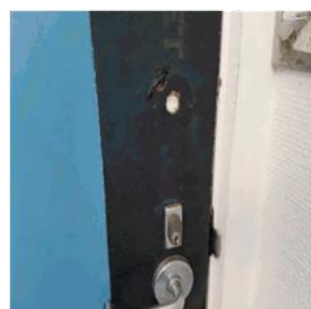
Figure 58: Failed finish to internal door
