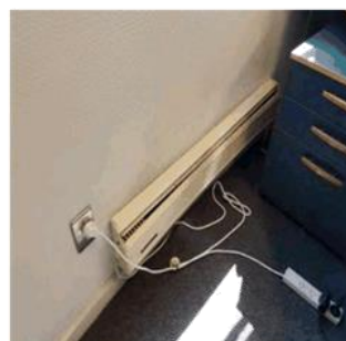
Figure 70: A typical Electric Wall heater as located to ground floor offices
