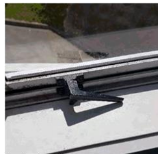
Figure 31: Window latch that is oxidising and framing that requires maintenance
