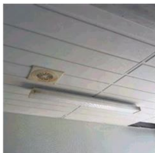
Figure 60: A typical Fluorescent batten light fitting
