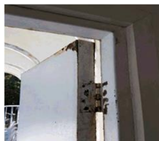
Figure 212: Failed hinges to media booth
