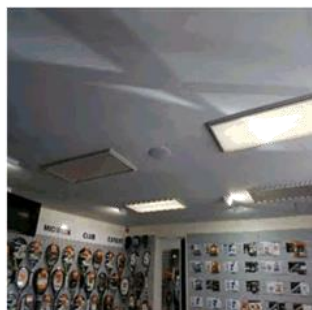
Figure 62: Recessed light fitting
