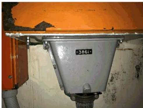
Photo – showing potential asbestos (white) sheet to bottom of switchboard cabinet
