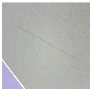
Figure 111: Cracking to court surface
