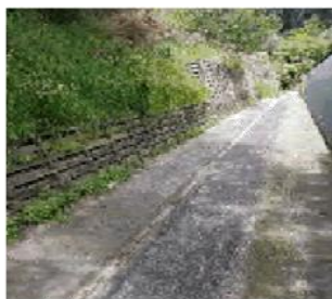
Figure 265: Timber retaining wall
