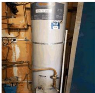
Figure 77: 160Ltr gas Hot water cylinder installed to the kitchen area
