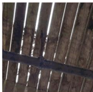
Figure 41: Gas pipe to building but bracket is rusting
