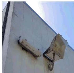
Figure 38: Rust to light housing and bracket and UV damage to the fitting cover
