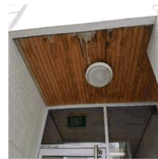
Figure 28: Varnished wooden Soffit to Eastern side door showing water staining
