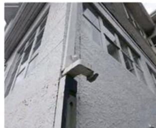
Figure 153: Failed UPVC downpipe system
