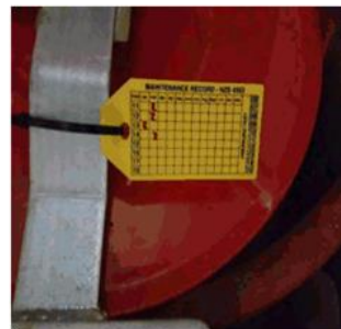
Figure 6: Yellow tag indicates the fire hose reel has not been serviced since 2014
