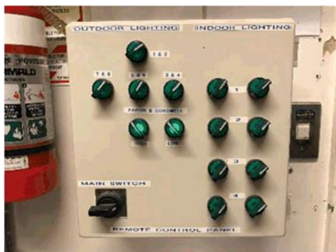
Photo – Court Lighting Remote Control Panel
