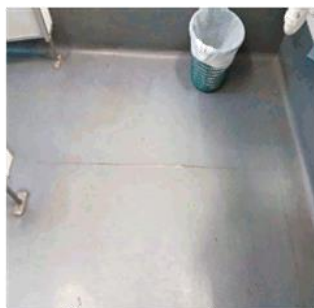
Figure 46: Vinyl to amenities is split and needs replacement
