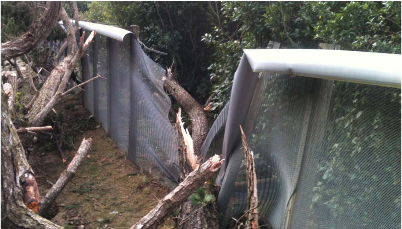
A major storm caused significant damage to our perimeter fence in June. Rob Masters.
