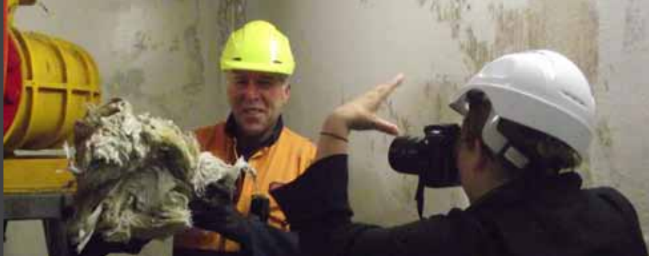
Hutt News reporter Karoline Tuckey grabs a picture of Hutt Valley Water Services' Steve Daken holding what's blocking the pumps at wastewater pumping stations.
