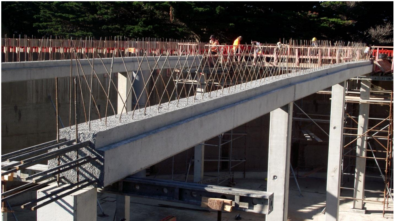
New beams form part of the strengthening measures put in place in Carmichael reservoir. This project was concluded in November 2012.
