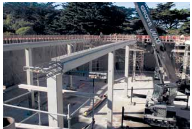
NEW COLUMNS AND ROOF BEAMS, ALONG WITH INTERNAL AND EXTERNAL RING BEAMS, ARE INSTALLED TO MAKE WELLINGTON'S CARMICHAEL RESERVOIR MORE EARTHQUAKE-RESISTANT.
