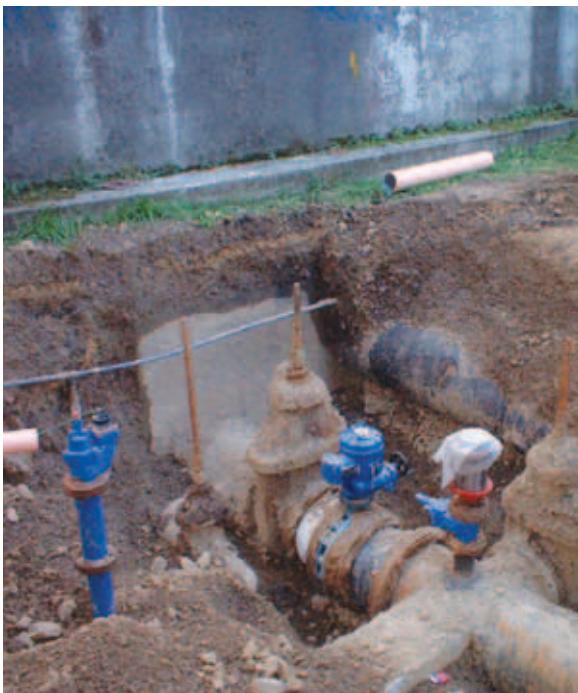
We systematically monitor city reservoirs for structural strength, and have nearly completed a programme of installing auto-shut-off valves with seismic couplings at major reservoirs. The valves ensure that a reservoir doesn’t lose all its water in the case of a sudden mains rupture in its supply zone.
