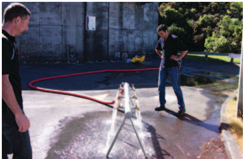
Chris Appleby (left) and Rob Jack check the distribution manifold at a Hutt City reservoir. These manifolds, which comprise several taps that can be fed directly from a reservoir, are installed at key locations in the region for use in an emergency event. They were recently put to use in Christchurch to help with the earthquake recovery.
