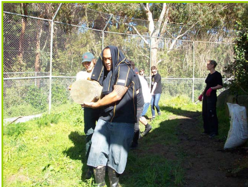
Neemia Tialata working on the new upgraded Lion enclosure
