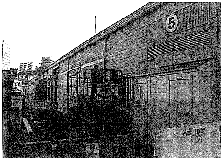
Repainting of Shed 5
