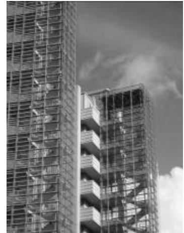
Sophisticated detailing in a contemporary building
