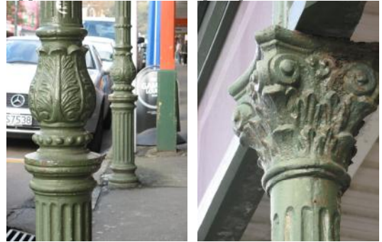
Detail of cast iron veranda posts
