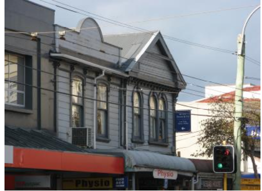
Upper level windows and parapets
