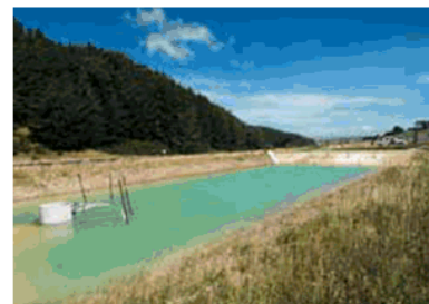
Above: Water then makes its way into the second pond, where sediment continues to settle before water is released into local gullies and streams.
