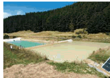
Above: Dirty water makes its way into the sediment-retention pond's first bay, where a coagulant is added to help settle sediment out of the water.
