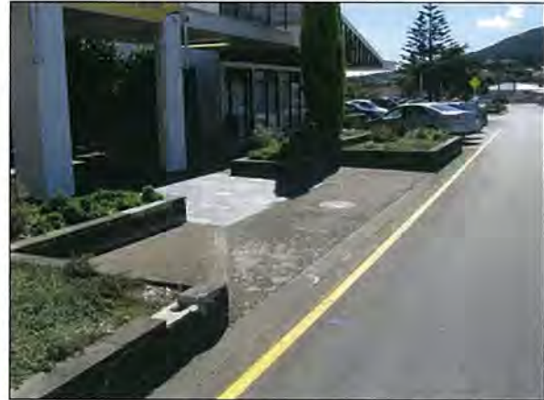
Non-compliant Southern Accessible Carpark (in front of council chambers)
