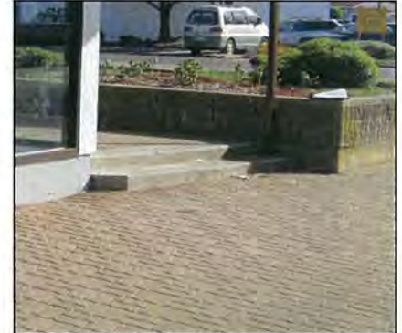
Community Hall - no ramp
