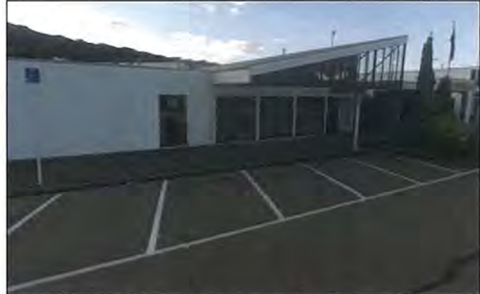
No kerb ramps present, Southern Side
