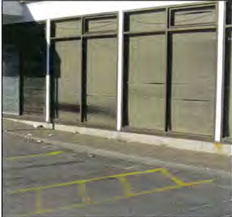
No kerb ramps present, East Side
