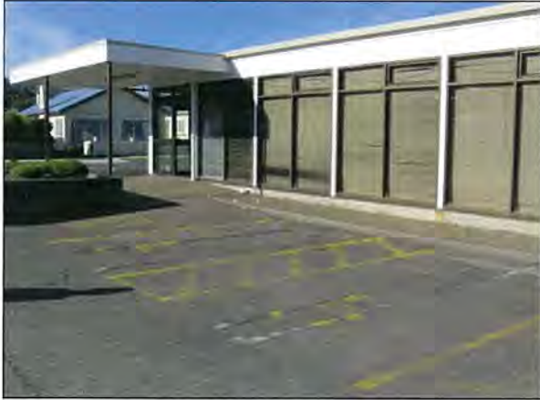
Existing accessible carparks (east)
