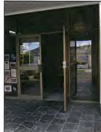
Front entrance doors
