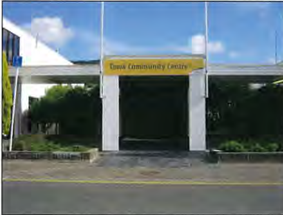
Poorly signed front entrance
