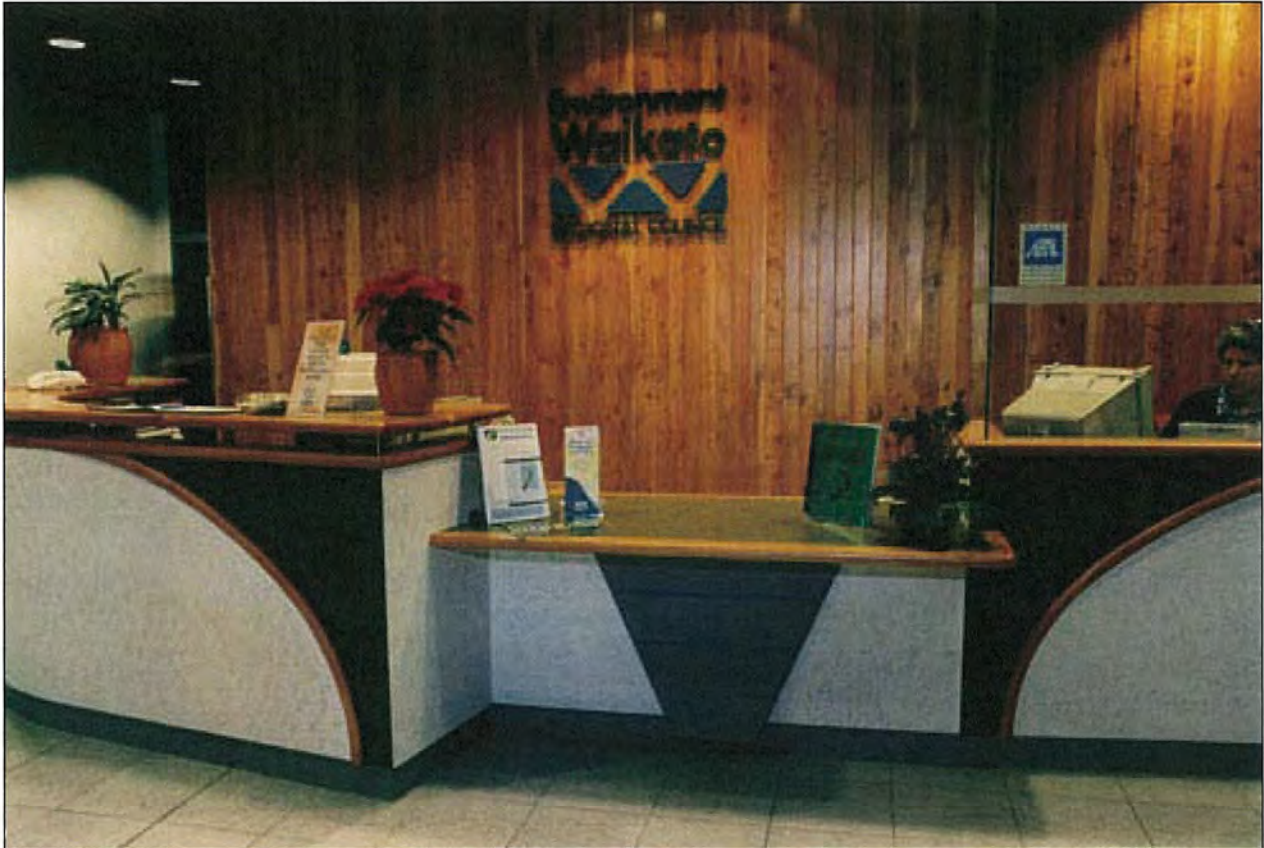
Example of a compliant accessible counter
