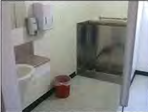
Male accessible toilets
