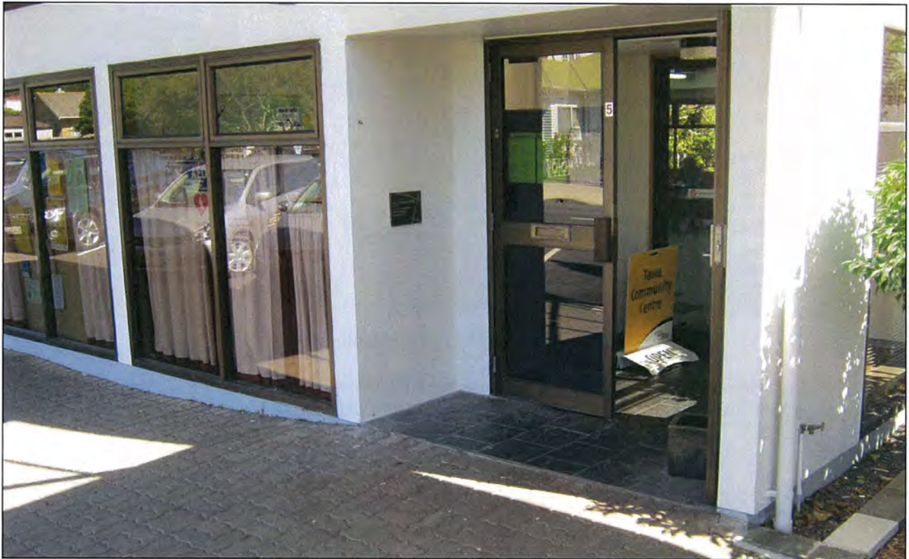
Front entrance to the Community Centre
