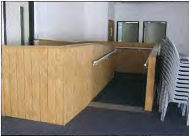
Ramp handrail projects into accessible route
