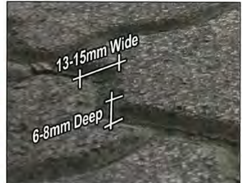
Zigzag brick pavers
