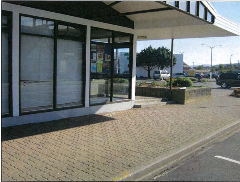
Existing steps in front of community hall entrance
