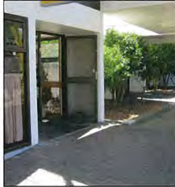
Community Centre ramp
