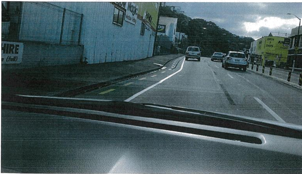
Kaiwharawhara corner – recent improvements made with road marking before, at and after the intersection are a good example of 1m cycle “lane” that has improved cycle safety and still room for 2 car lanes
