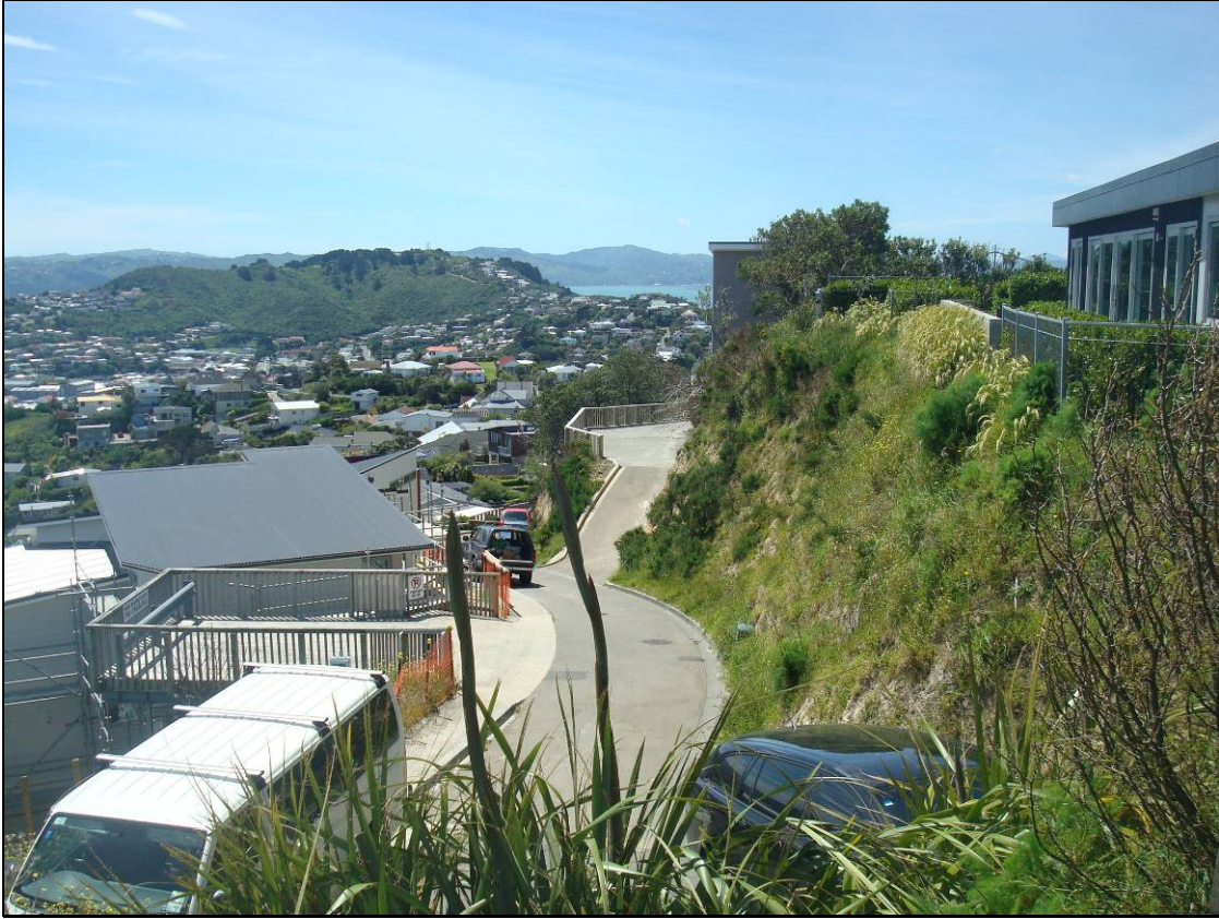
Beside reservoir structure, looking north.
