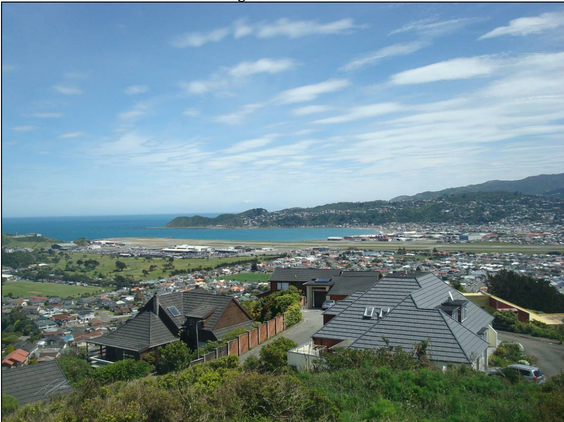
Beside reservoir structure, looking south-west.
